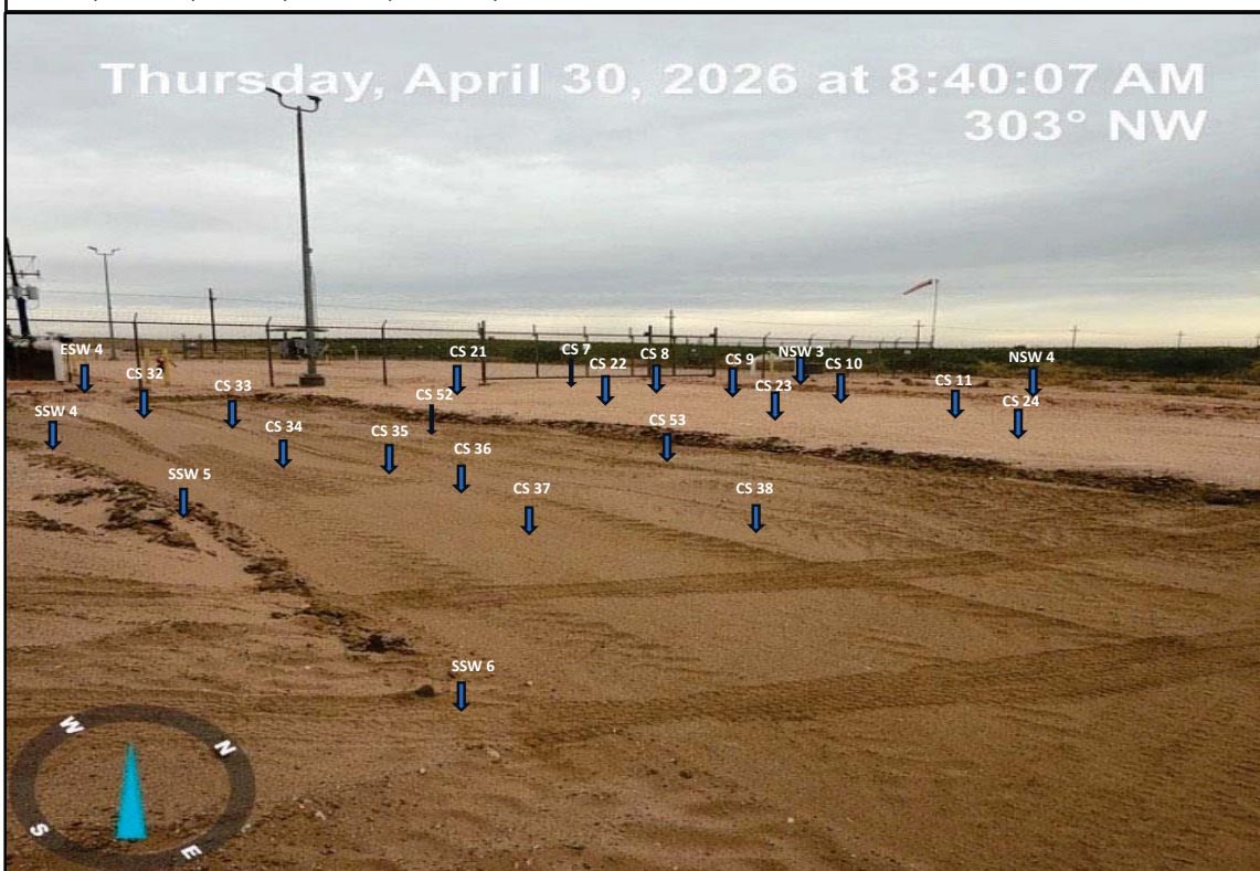
View Northwest - Remediation activities (i.e., excavation and stockpiling of impacted material) ongoing. Sample locations CS 7 thru CS 11, CS 21 thru CS 24, CS 32 thru CS 38, CS 52, CS 53, NSW 3, NSW 4, and ESW 4 are shown.
