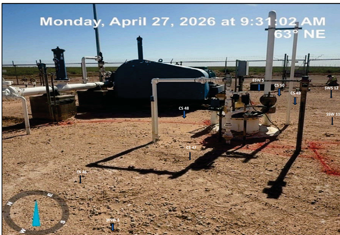
View Northeast - Remediation activities (i.e., excavation and stockpiling of impacted material) ongoing. Sample locations CS 46 thru CS 50 and ESW 5, SWS 11, SWS 12, and WSW 5 are shown.
