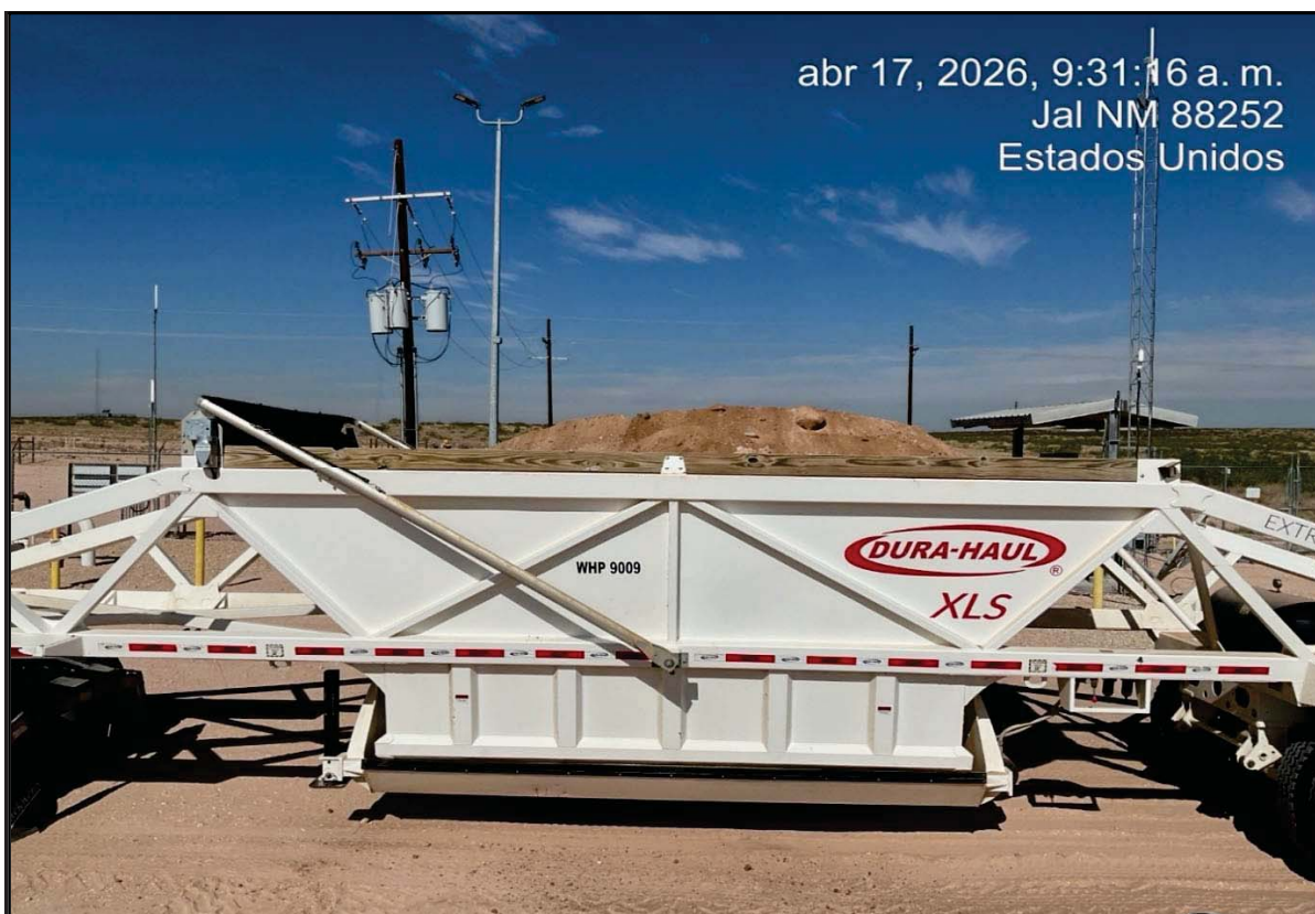
View West - Exporting excavated impacted material offsite to an approved disposal.
