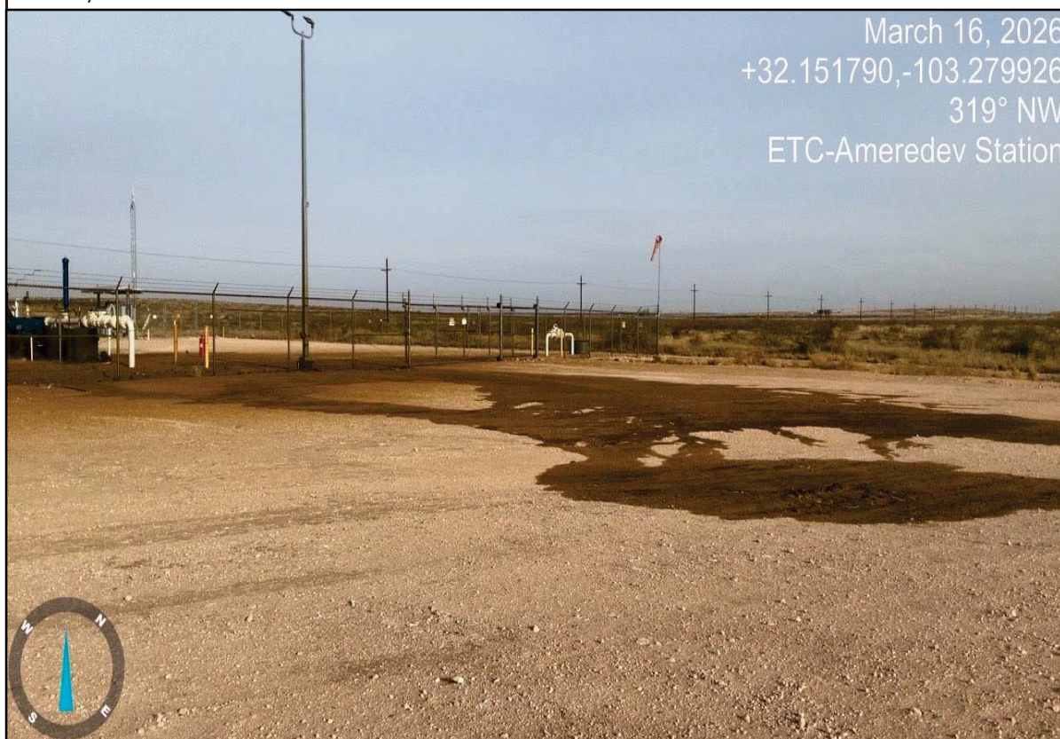
View Northwest - A portion of the release footprint (i.e., dark stained surface middle of photograph).
