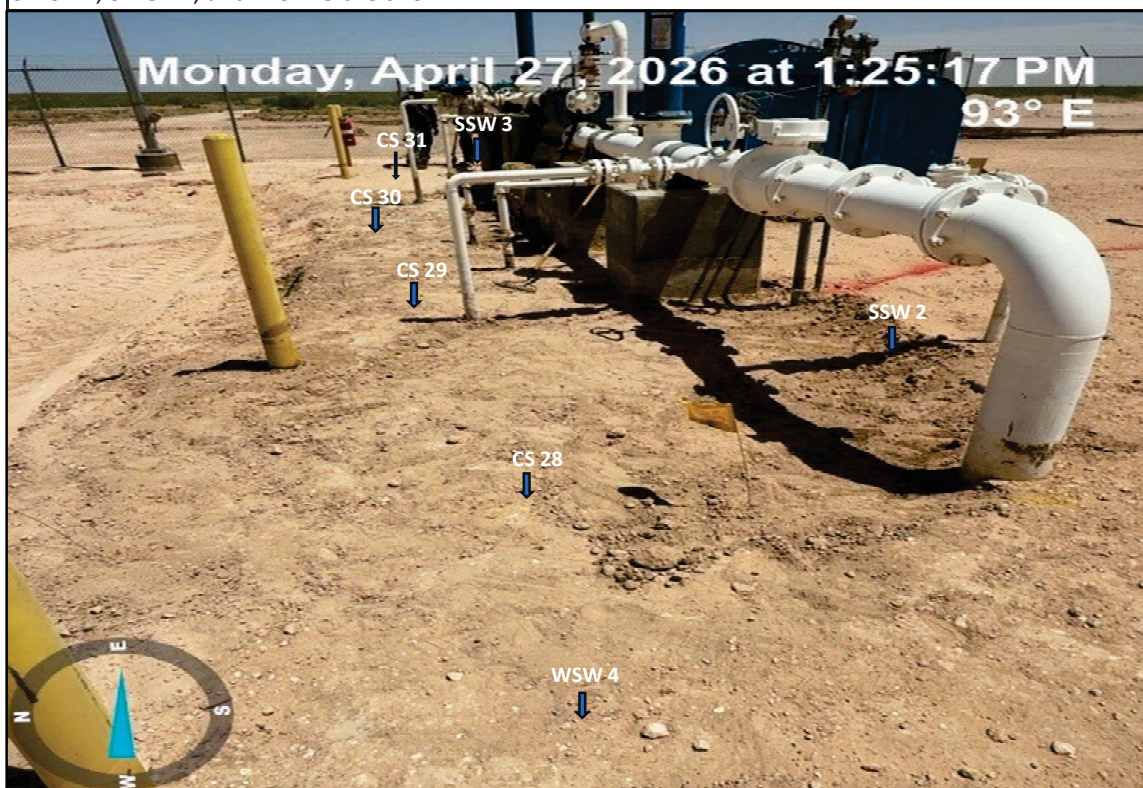
View East - Remediation activities (i.e., excavation and stockpiling of impacted material) ongoing. Sample locations CS 28 thru CS 31 and SWS 2, SWS 3, and WSW 4 are shown.
