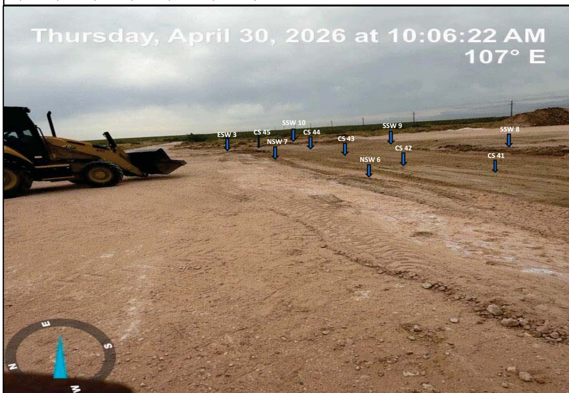
View East - Remediation activities (i.e., excavation and stockpiling of impacted material) ongoing. Sample locations CS 41 thru CS 45, NSW 6, NSW 7, ESW 3, SSW 8, and SSW 9 are shown.
