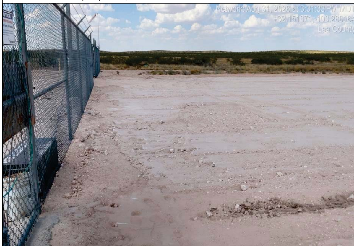
View West - Remediation activities (i.e., backfilling and surface contouring within the release footprint) is complete.
