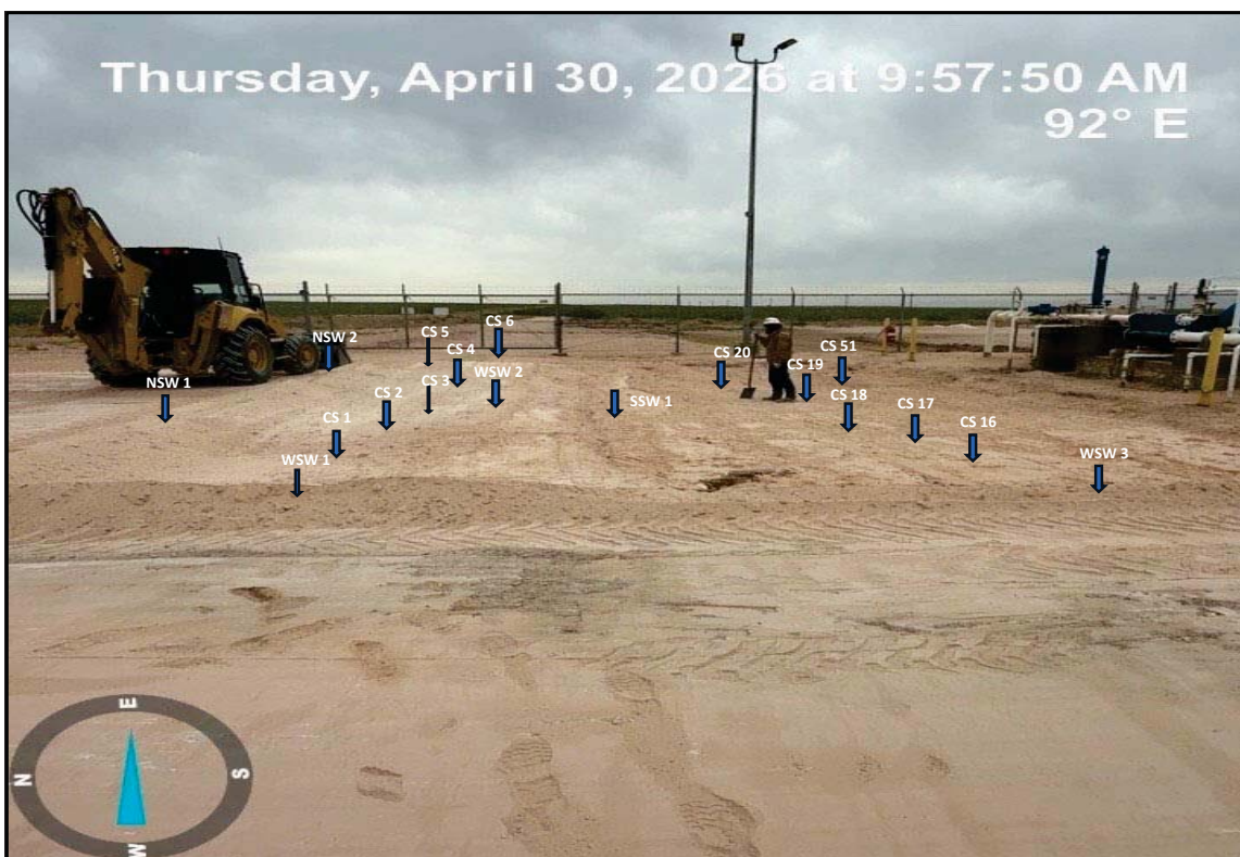
View East - Remediation activities (i.e., excavation and stockpiling of impacted material) ongoing. Sample locations CS 1 thru CS 6, CS 16 thru CS 20, CS 51, NSW 1, NSW 2, SSW 1, WSW 1, WSW 2, and WSW 3 are shown.
