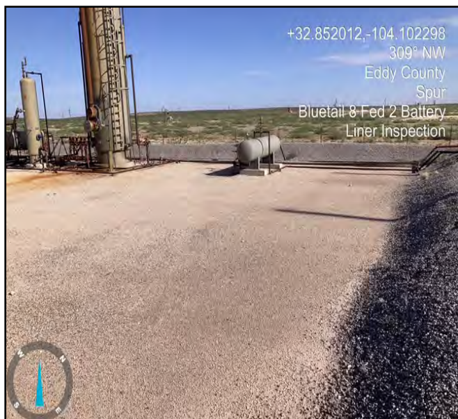
Photograph taken during liner inspection facing northwest.
