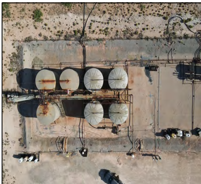
Aerial photo taken during liner inspection.
