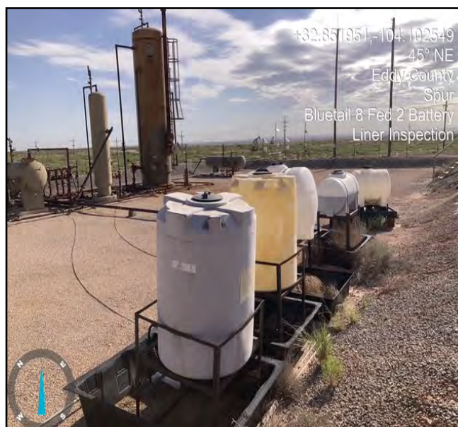
Photograph taken during liner inspection facing northeast.
