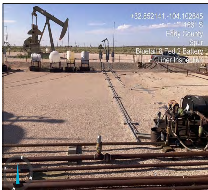
Photograph taken during liner inspection facing south.
