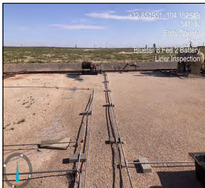
Photograph taken during liner inspection facing north.
