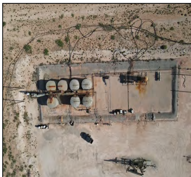
Aerial photo taken during liner inspection.
