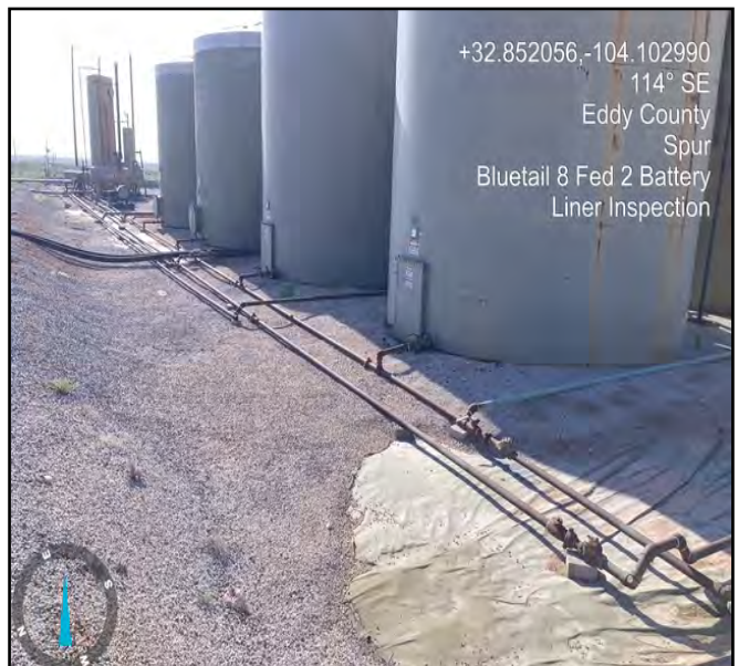
Photograph taken during liner inspection facing southeast.
