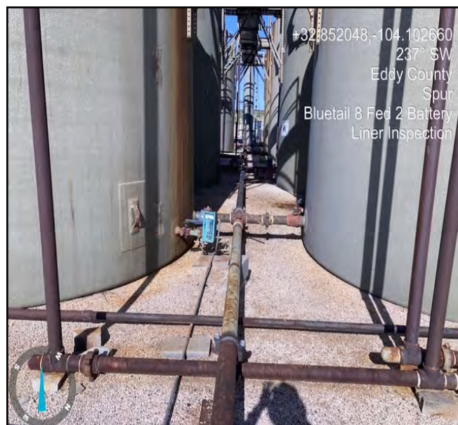
Photograph taken during liner inspection facing southwest.
