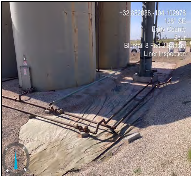
Photograph taken during liner inspection facing southeast.
