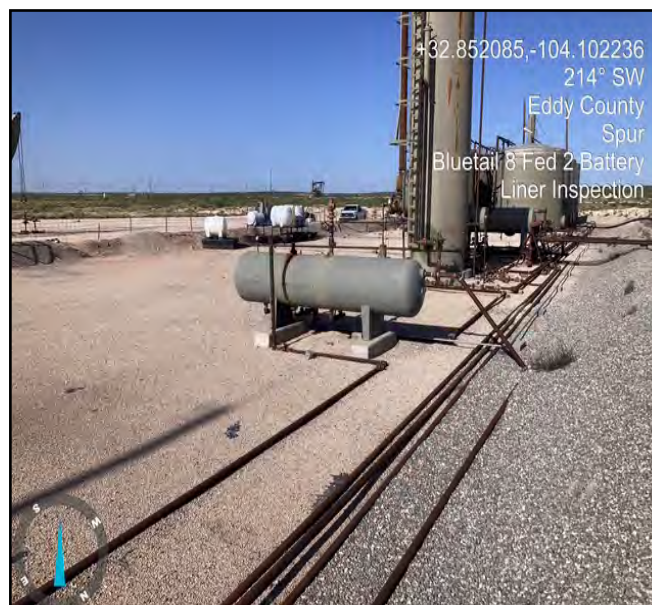
Photograph taken during liner inspection facing southwest.
