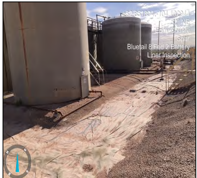
Photograph taken during liner inspection facing northeast.
