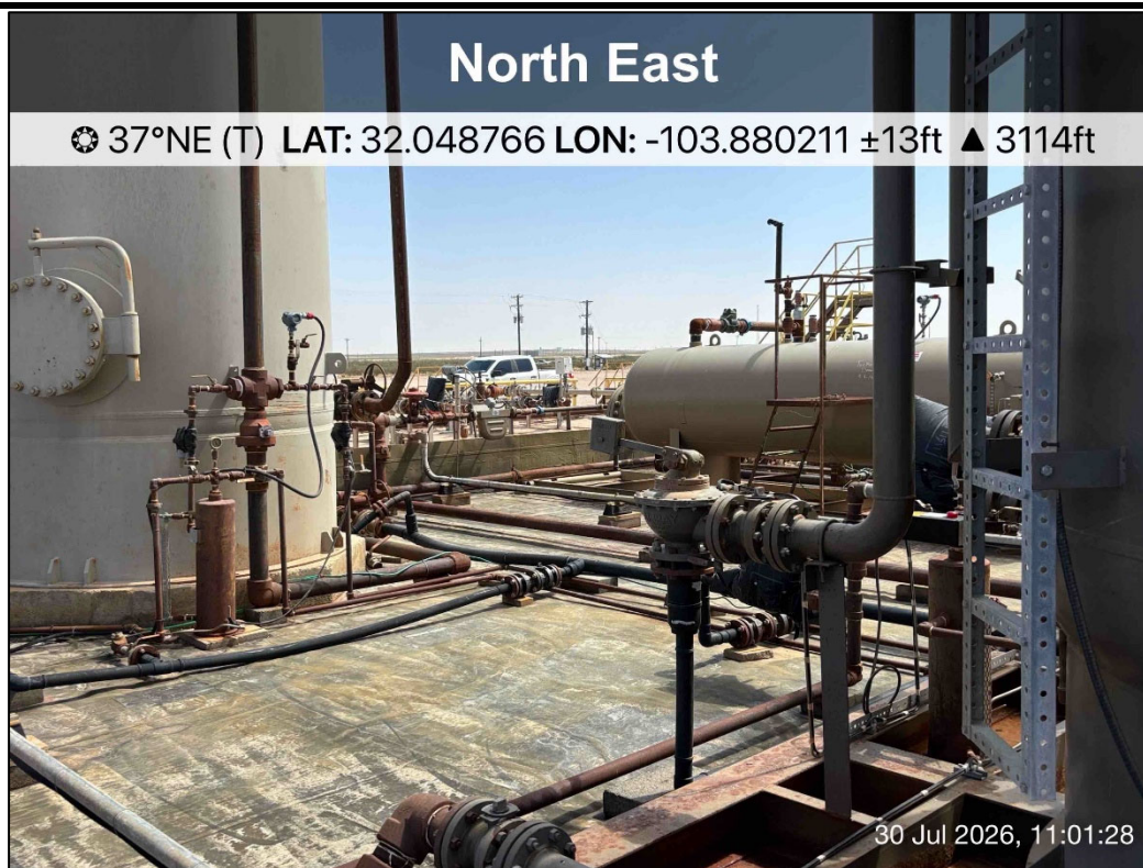
PHOTO 11: Northeastern view during liner inspection activities. 7/30/2026
