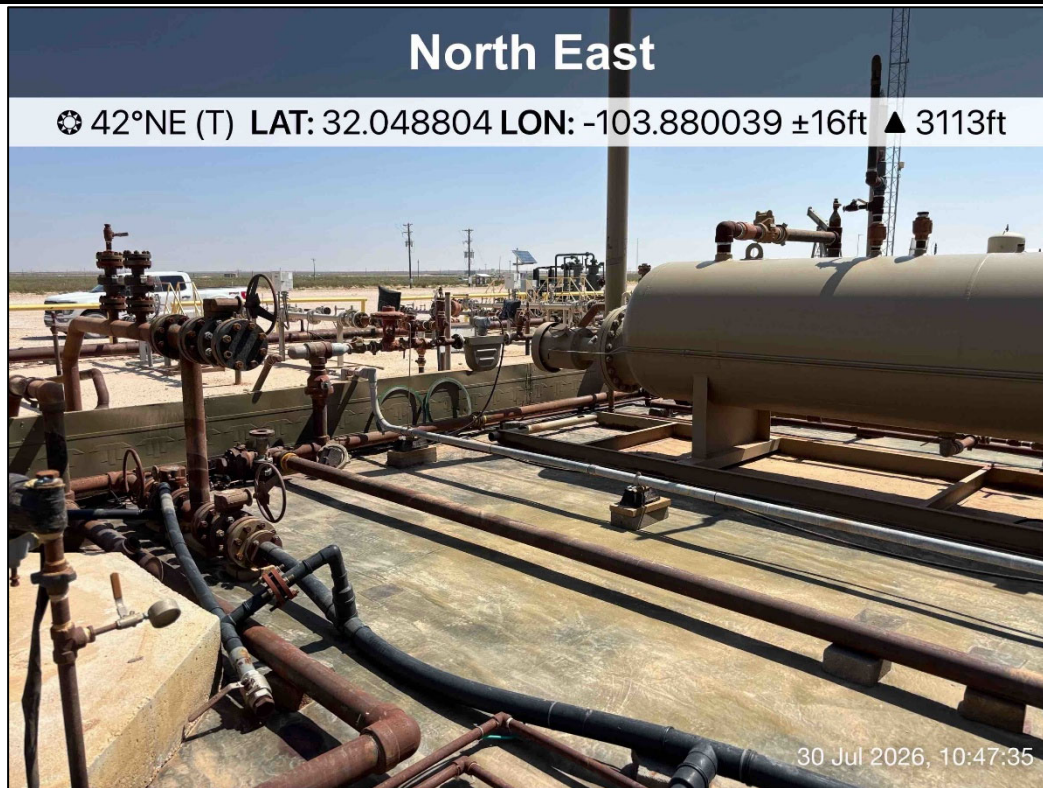
PHOTO 23: Northeastern view during liner inspection activities. 7/30/2026
