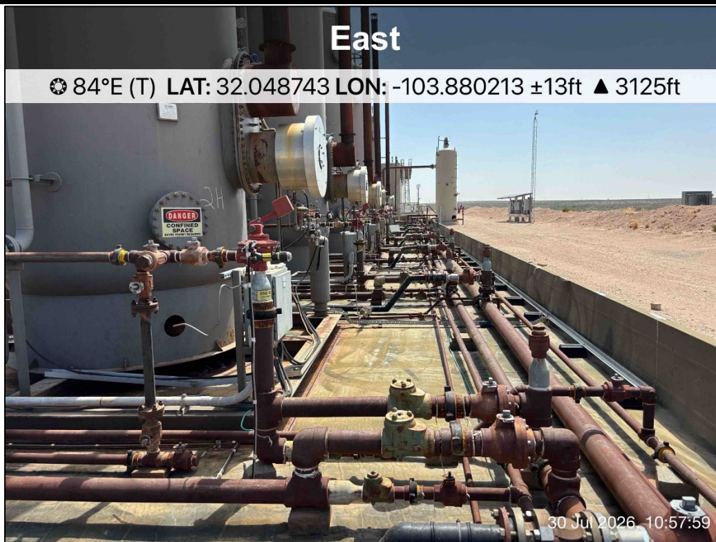
PHOTO 17: Eastern view during liner inspection activities. 7/30/2026
