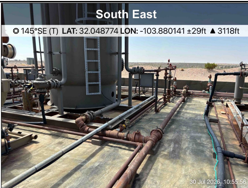
PHOTO 18: Southeastern view during liner inspection activities. 7/30/2026
