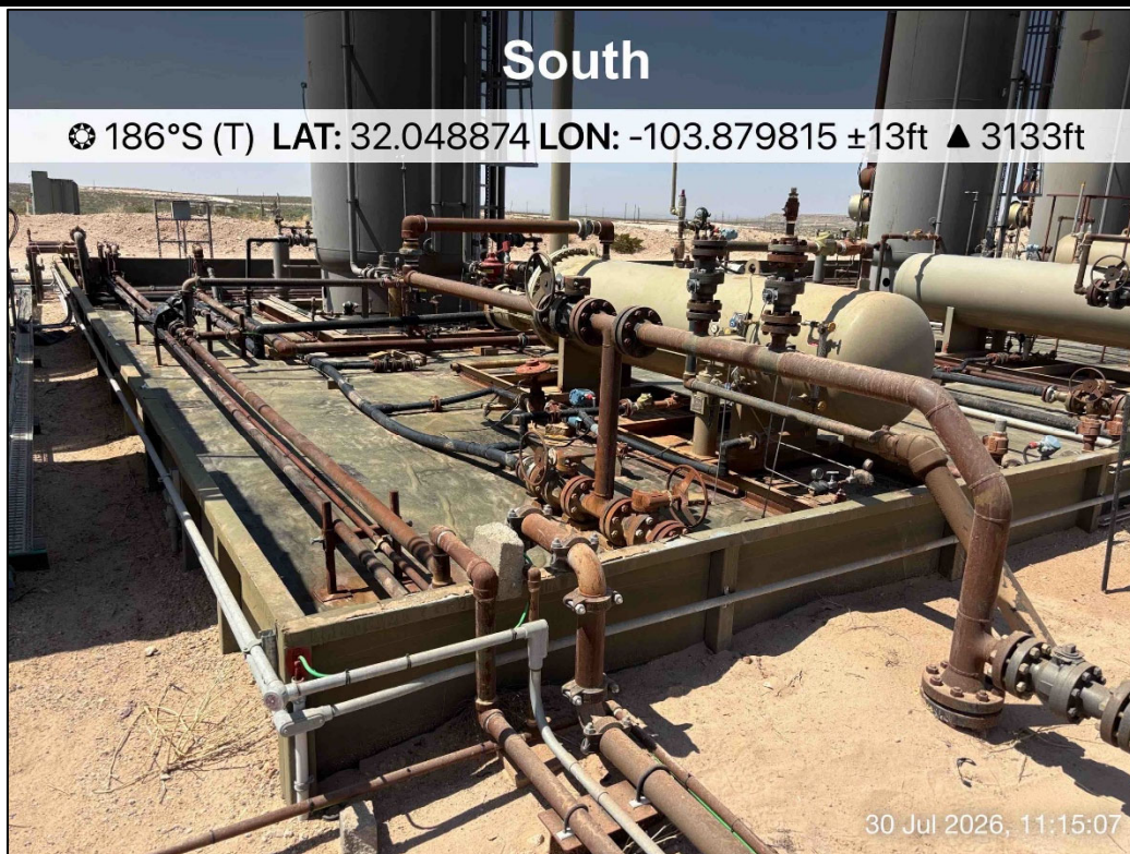
PHOTO 6: Southern view outside of containment during liner inspection activities. 7/30/2026
