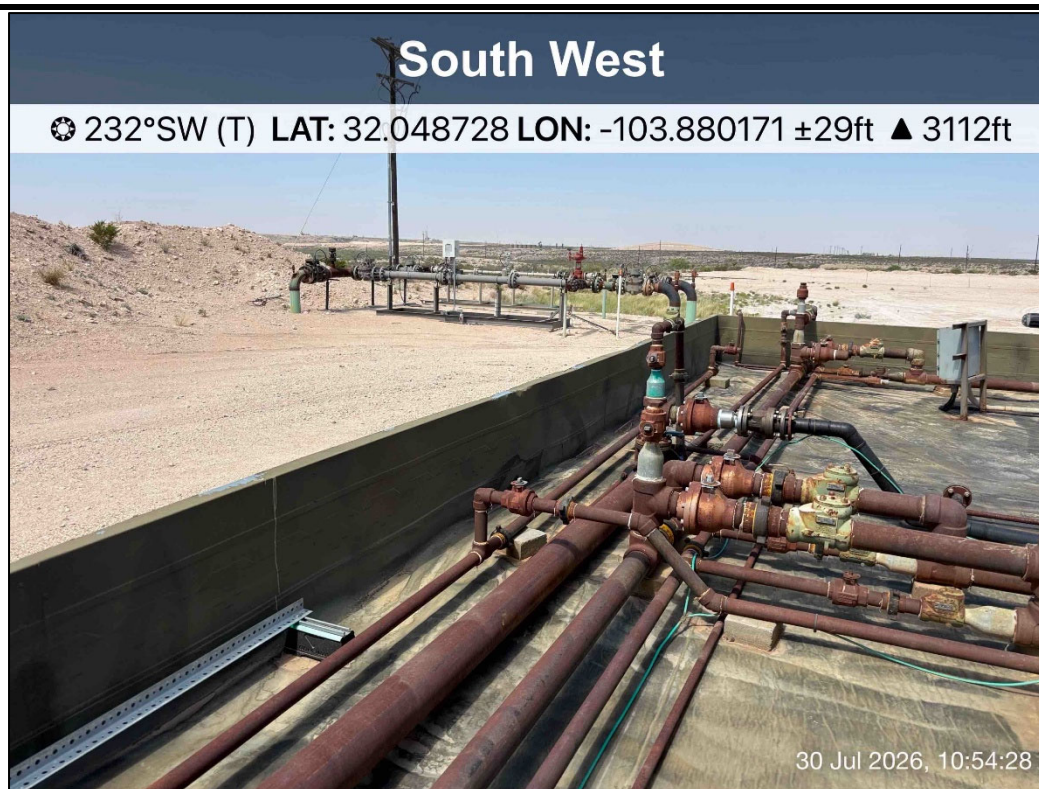
PHOTO 20: Southwestern view during liner inspection activities. 7/30/2026
