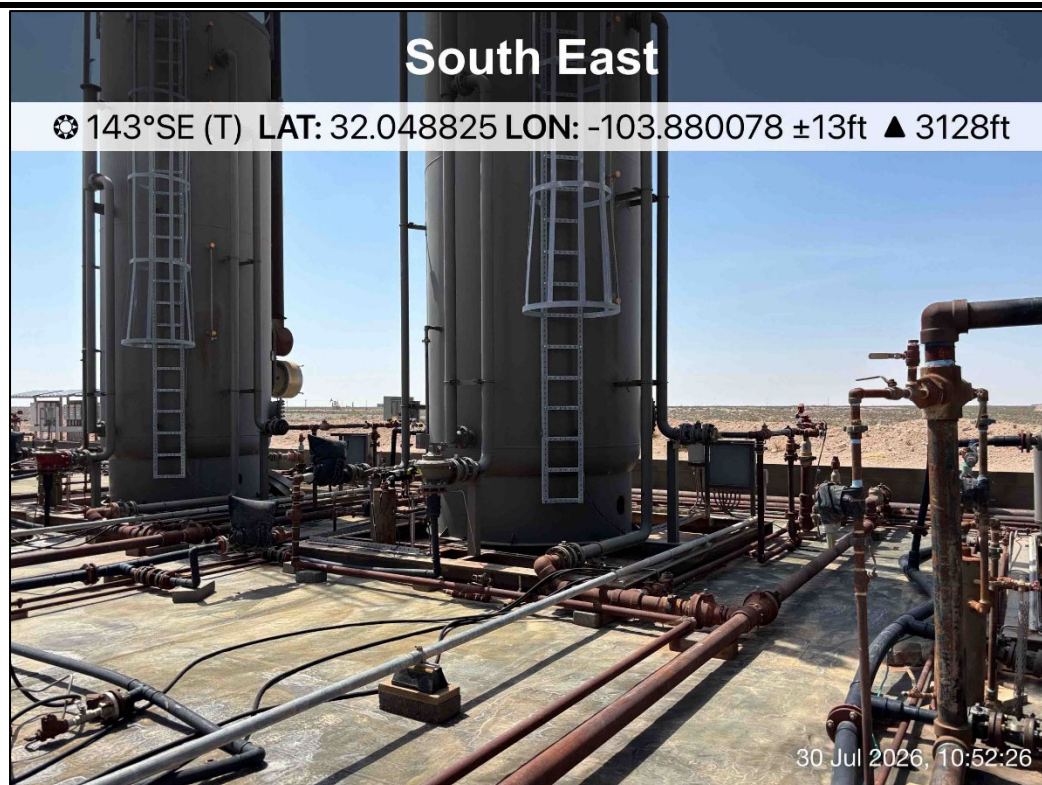
PHOTO 22: Southeastern view during liner inspection activities. 7/30/2026
