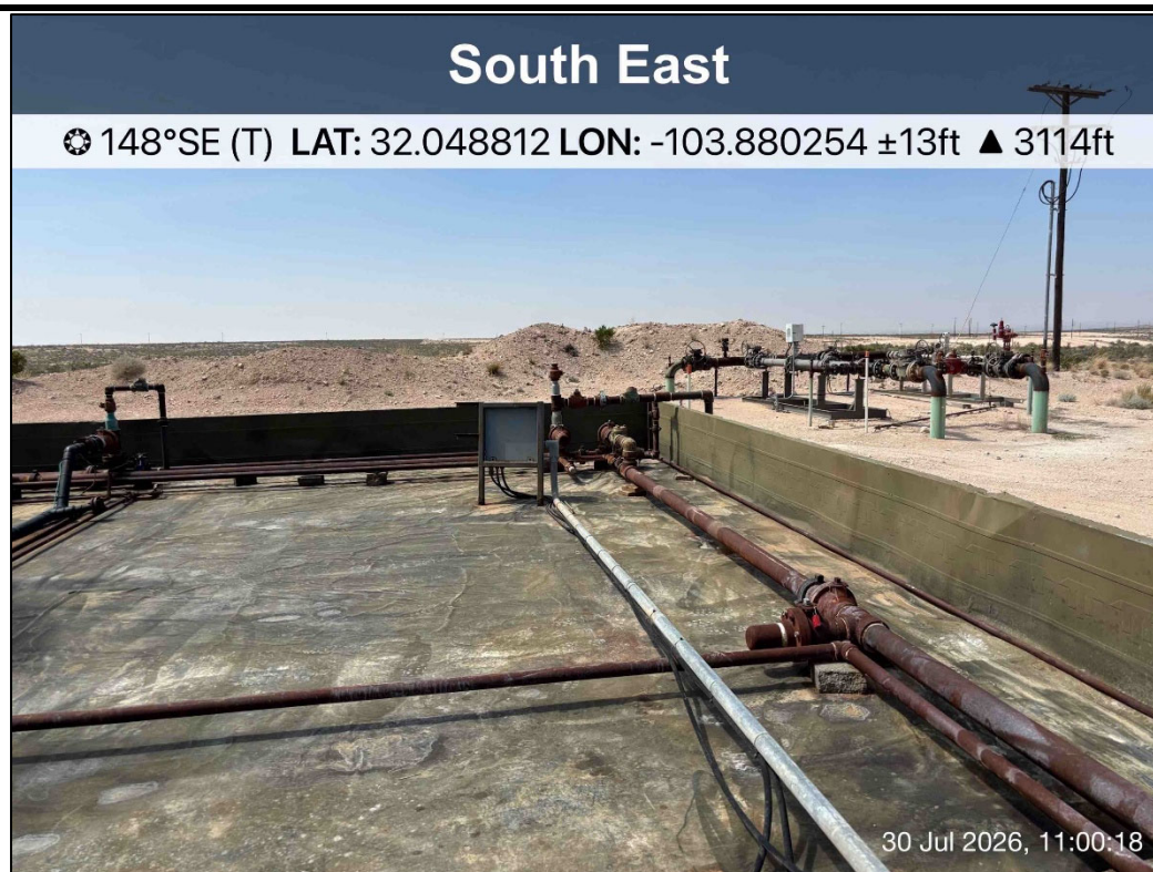
PHOTO 12: Southeastern view during liner inspection activities. 7/30/2026
