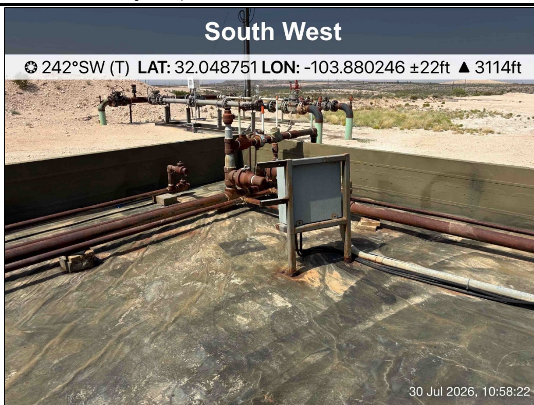
PHOTO 16: Southwestern view tanks during liner inspection activities. 7/30/2026
