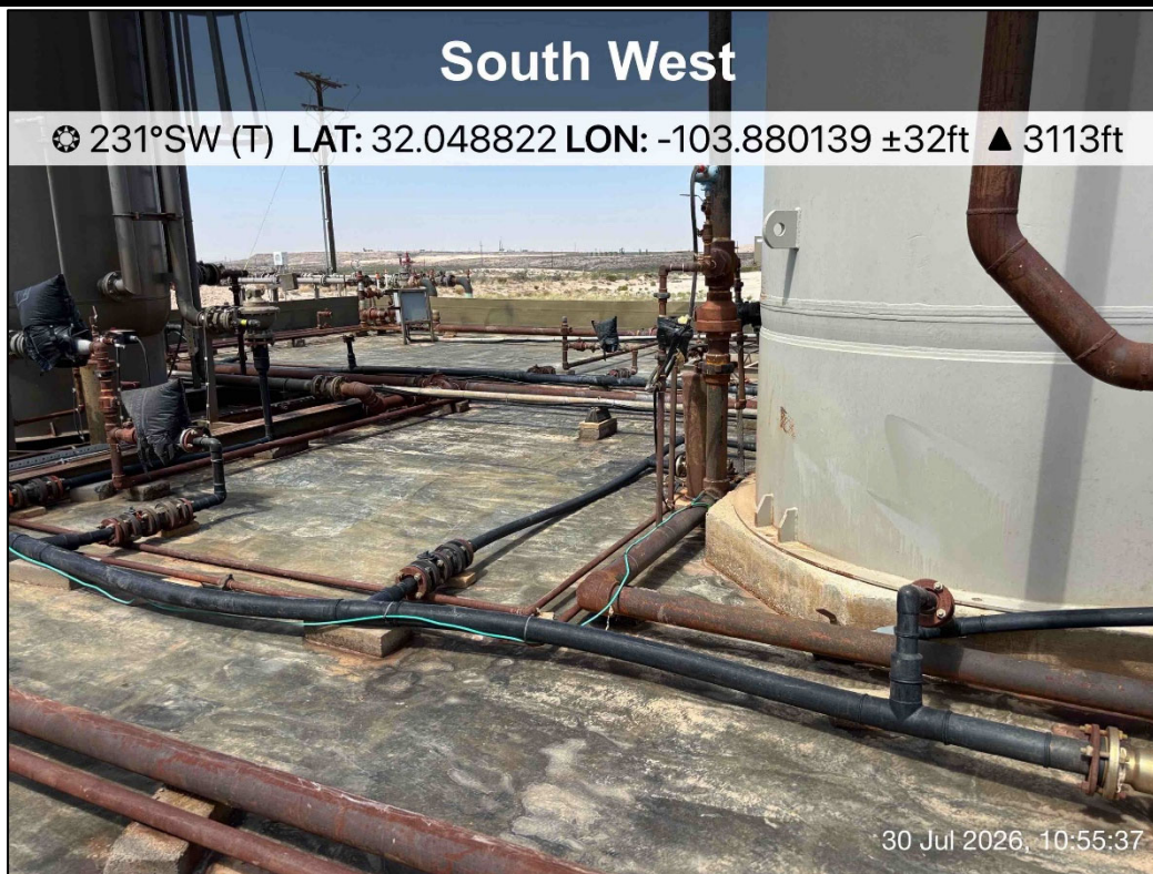
PHOTO 19: Southwestern view during liner inspection activities. 7/30/2026
