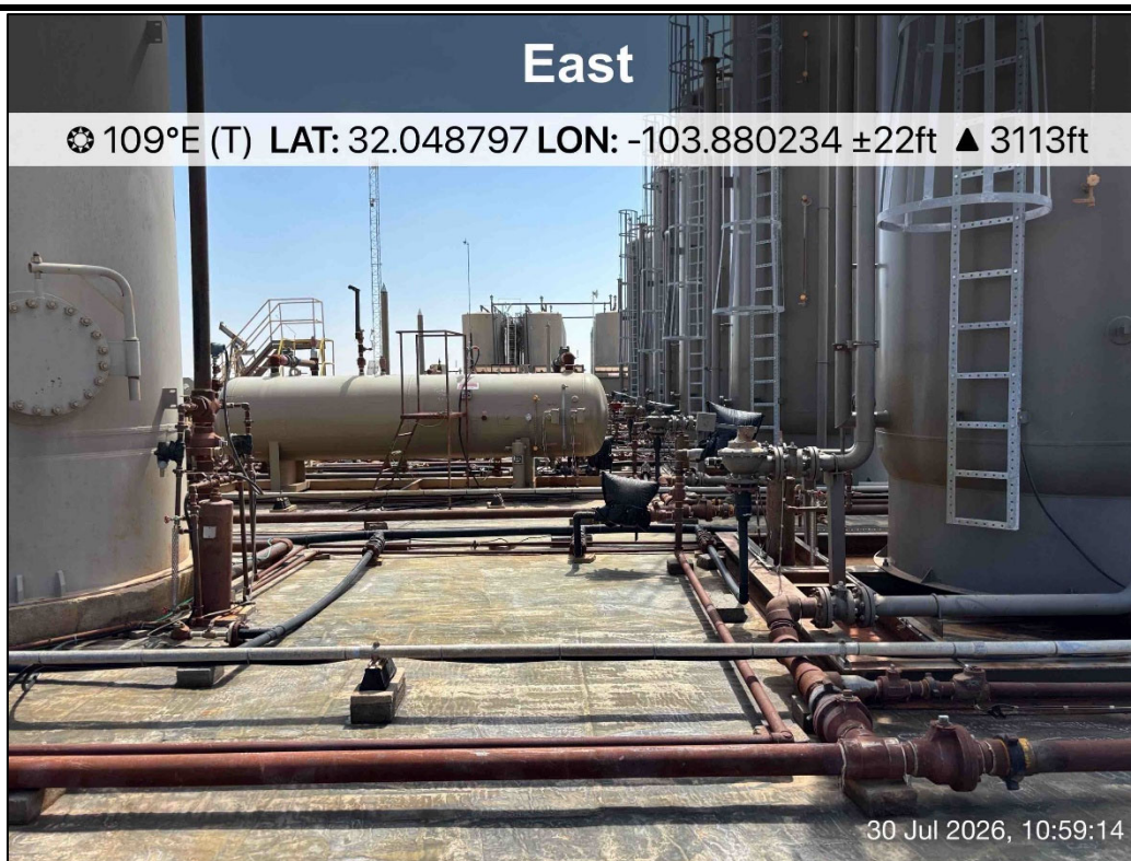
PHOTO 14: Eastern view during liner inspection activities. 7/30/2026
