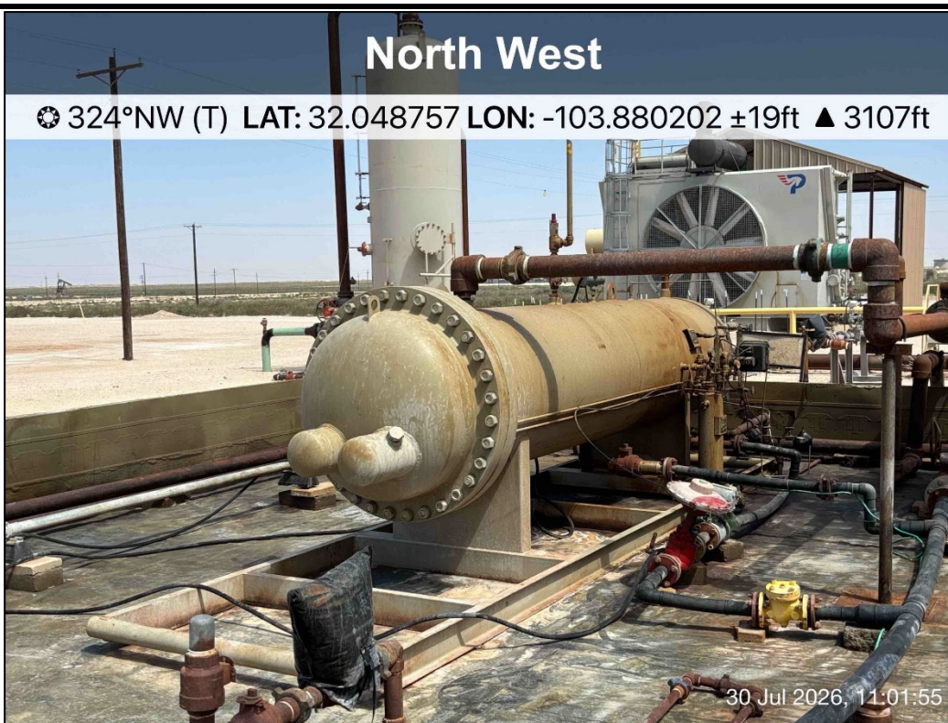
PHOTO 10: Northwestern view during liner inspection activities. 7/30/2026
