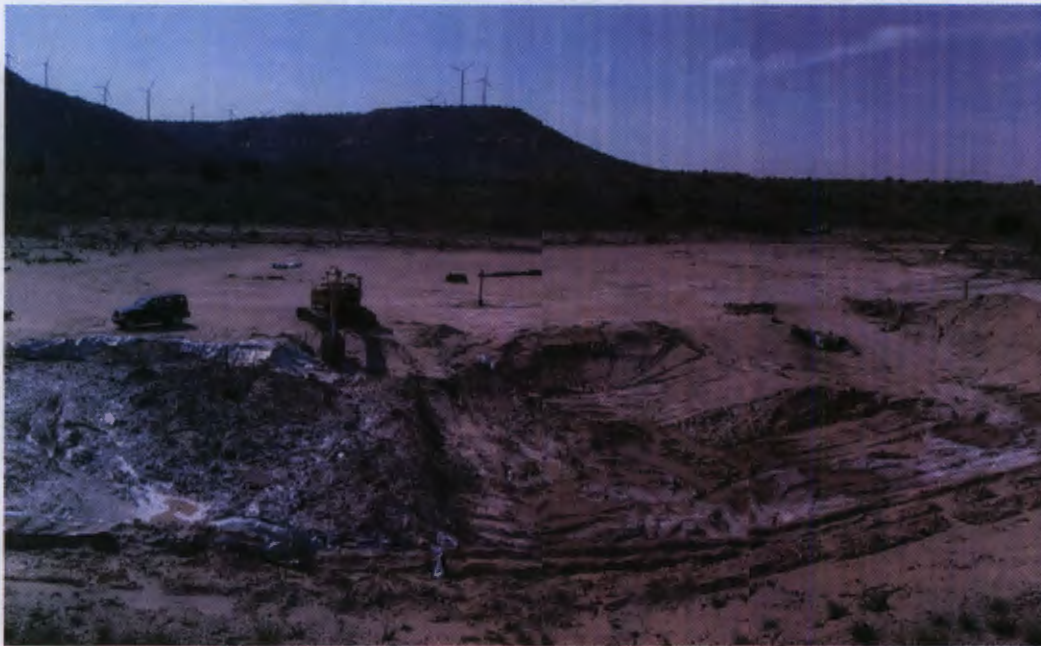
Figure 1: Looking to the west. Materials are being moved from the temporary drilling pit on the north (right) to the burial trench on the south (left).
