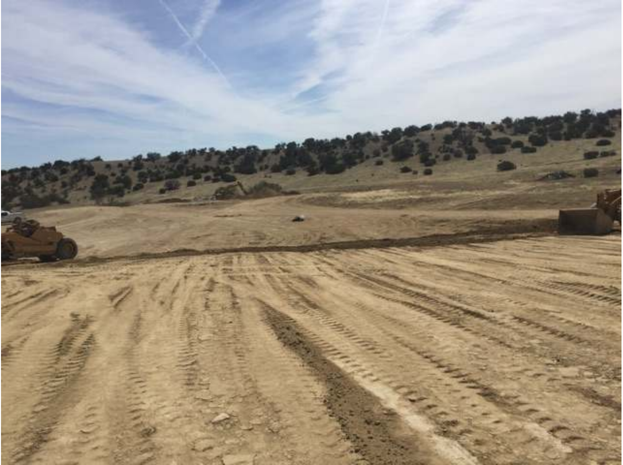
Interim reclamation of lined burial trench and CC14X temporary drilling pit areas.
