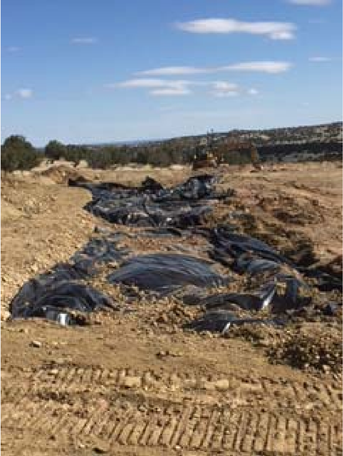
Outer edges of trench liner folded over waste material prior to installation of geomembrane cover.
