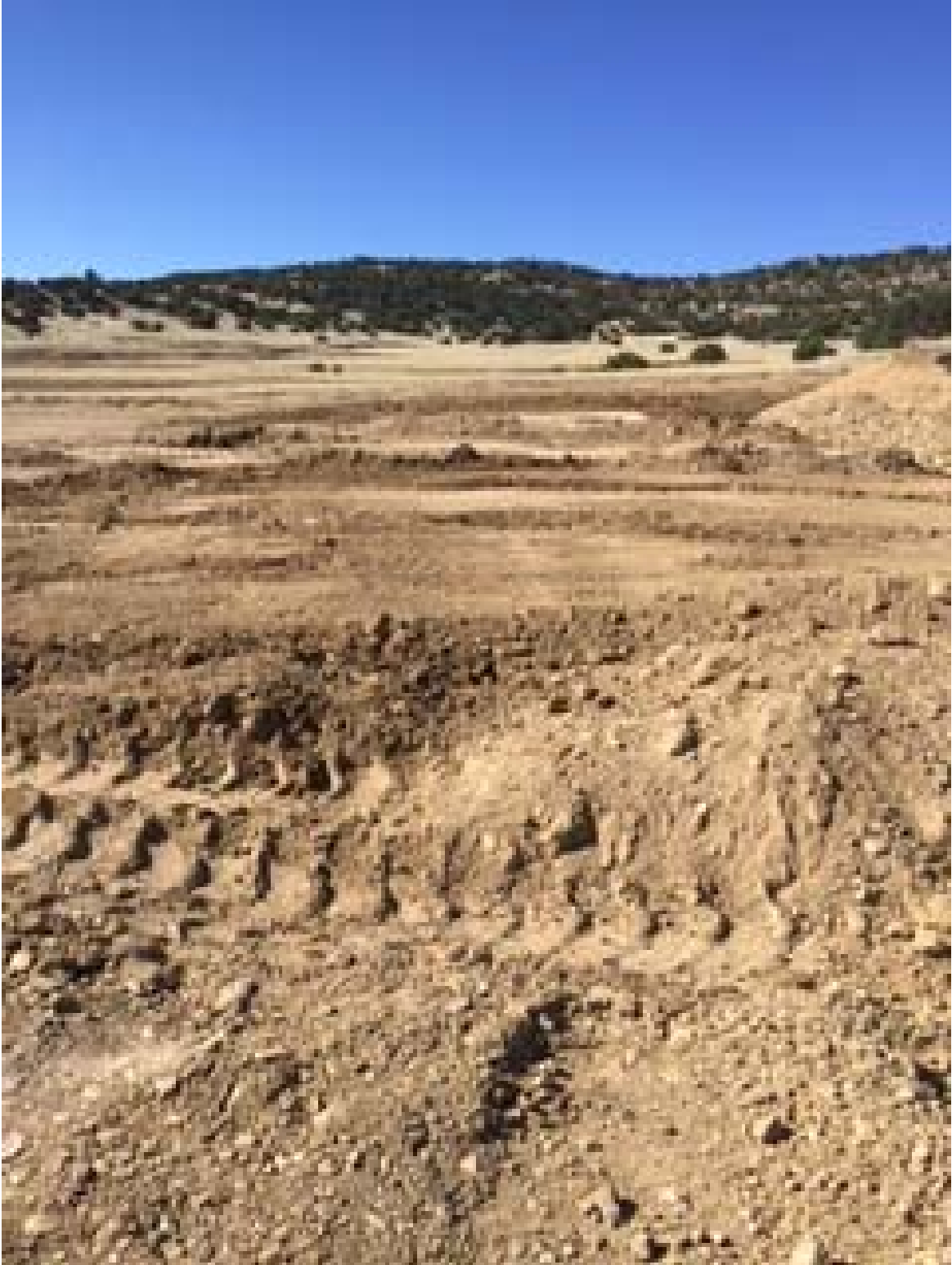
Soil cover being placed over lined burial trench.
