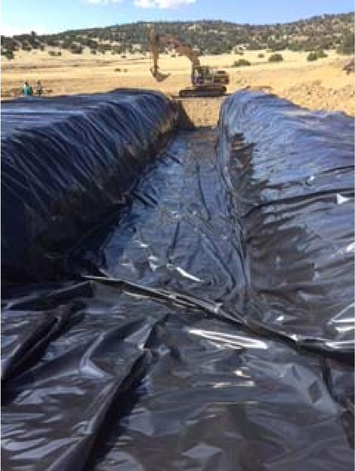
Installation of 30 mil LLDPE liner in burial trench excavation.
