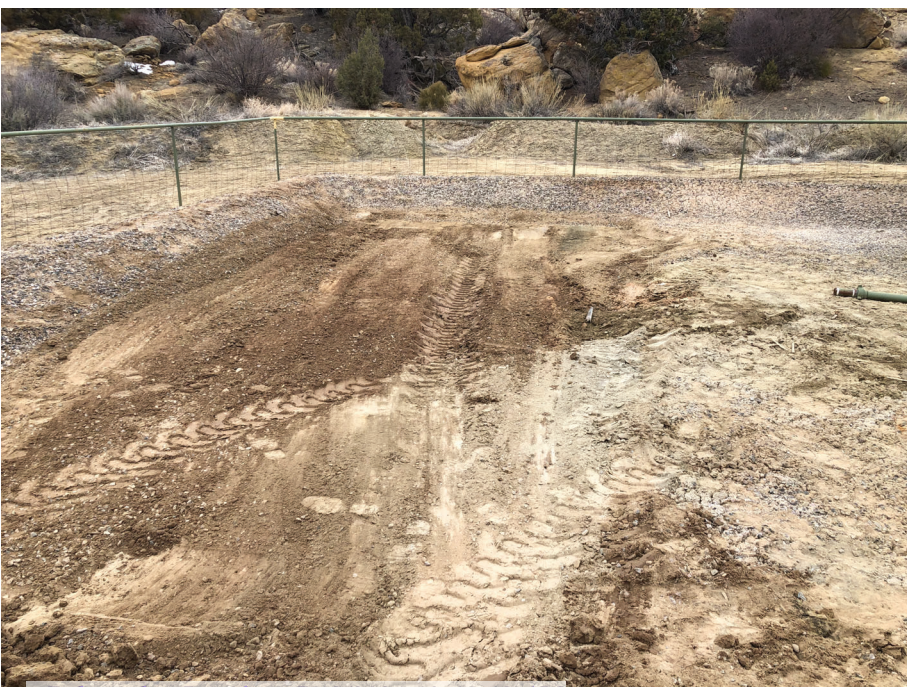
Area of 21 bbl tank backfilled
