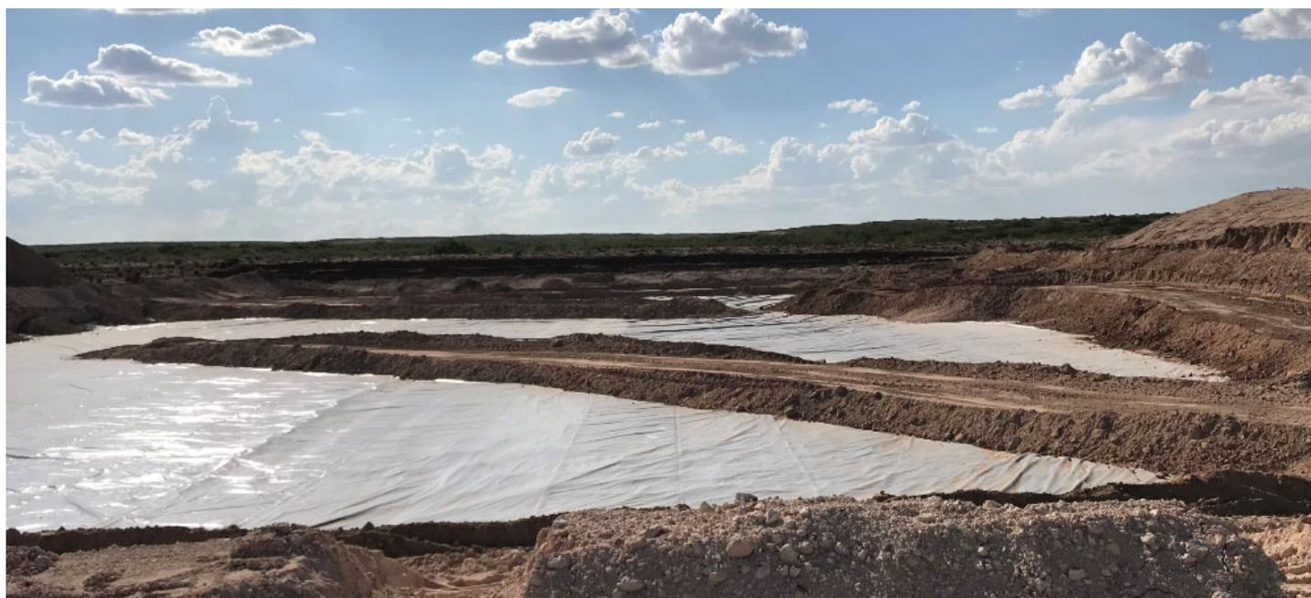
Figure 4 - Liner Placement (9/26/19)
