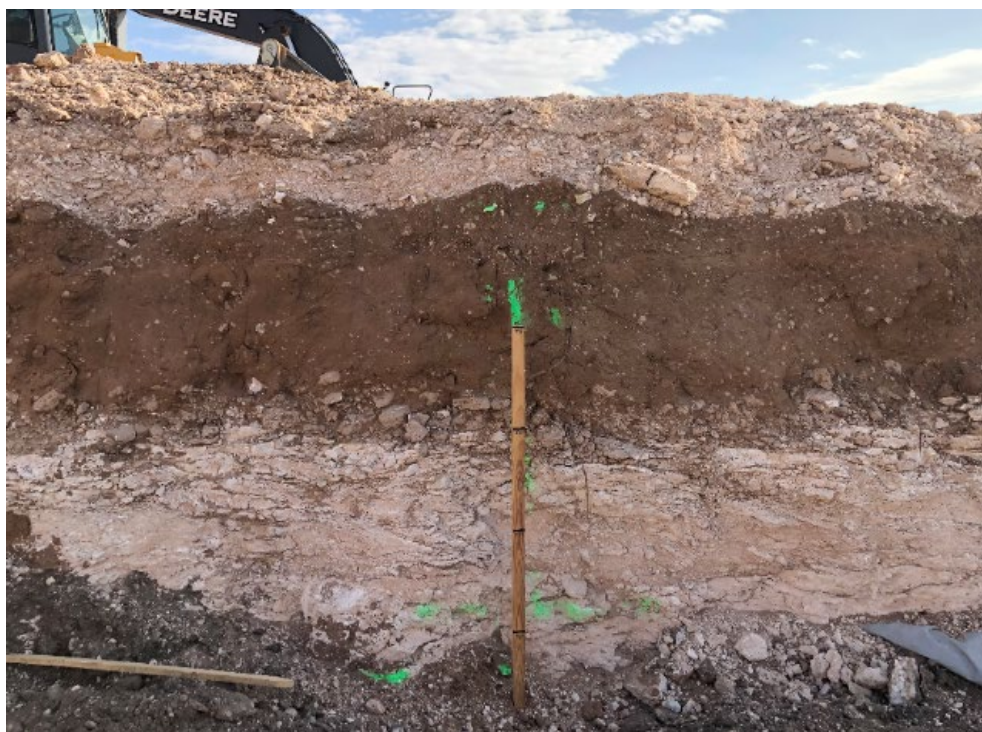
Figure 5 - Reclaimed surface is a minimum of 4 feet below natural ground.
