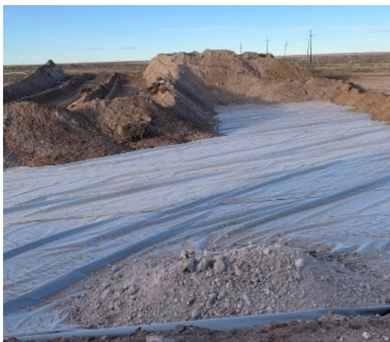
Figure 6 - Liner placement (12/16/19)
