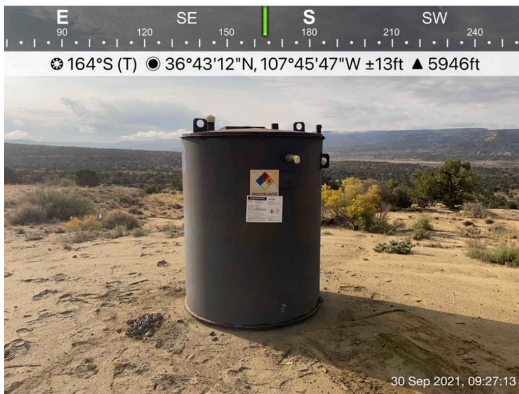
Photo 2: 21 bbls steel tank "B" prior to removal, 9/30/21.
