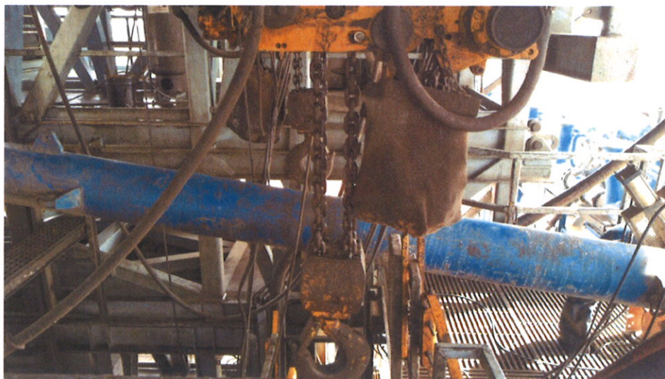
Figure 2: BOP Winch System
