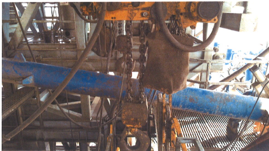
Figure 2: BOP Winch System
