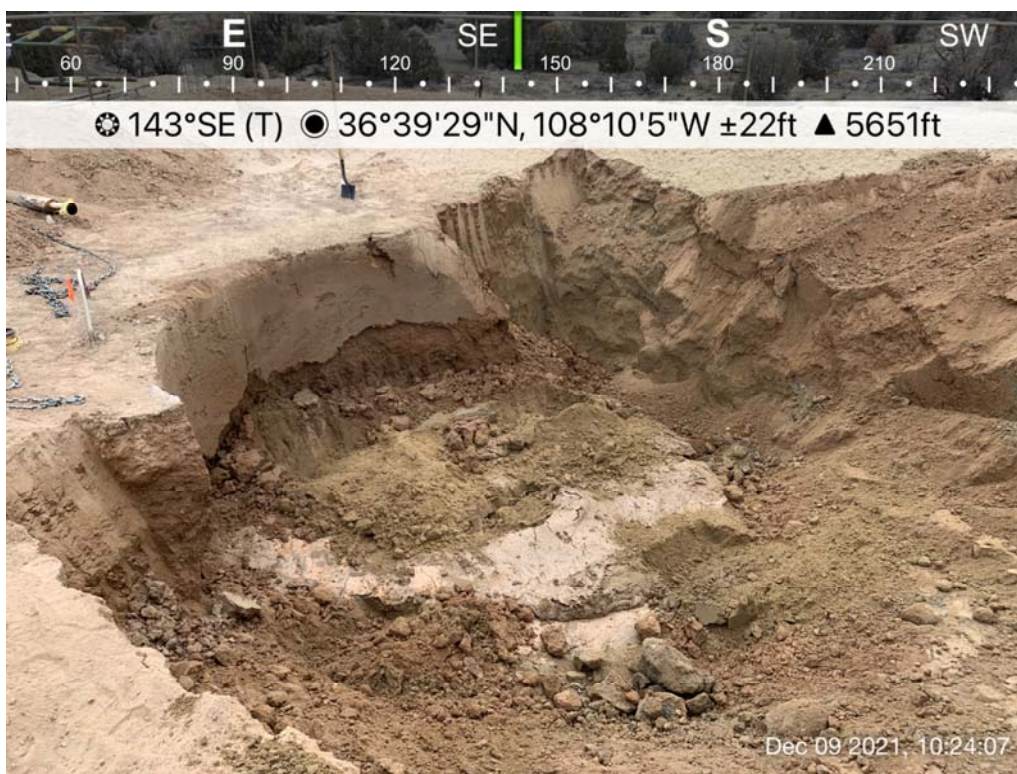
Photo 3: Former location of 95 bbls steel tank “A” following removal, 12/9/21.
