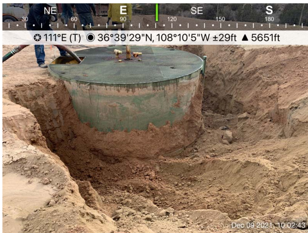
Photo 2: 95 bbls steel tank "A" during removal, 12/9/21.
