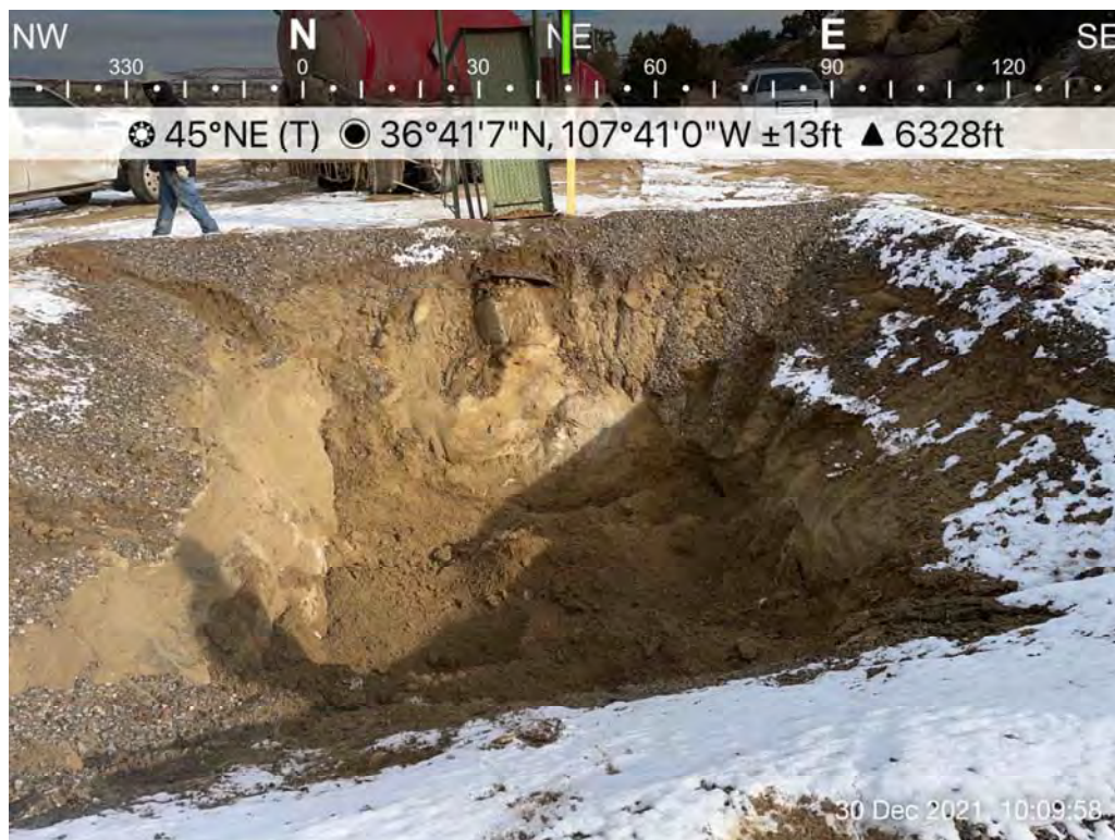
Photo 3: Former location of 45 bbls steel tank "A" following removal, 12/30/21.
