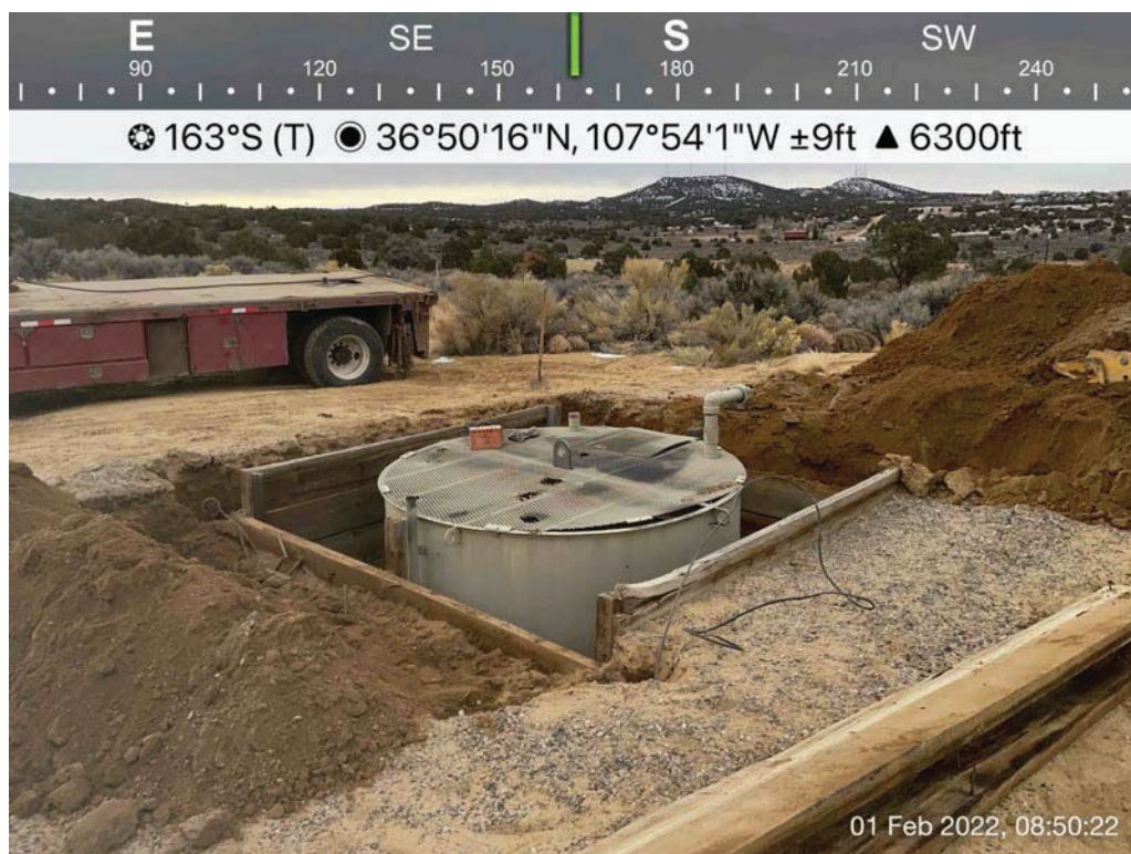
Photo 2: 45 bbls steel tank "A" prior to removal, 2/1/2022.
