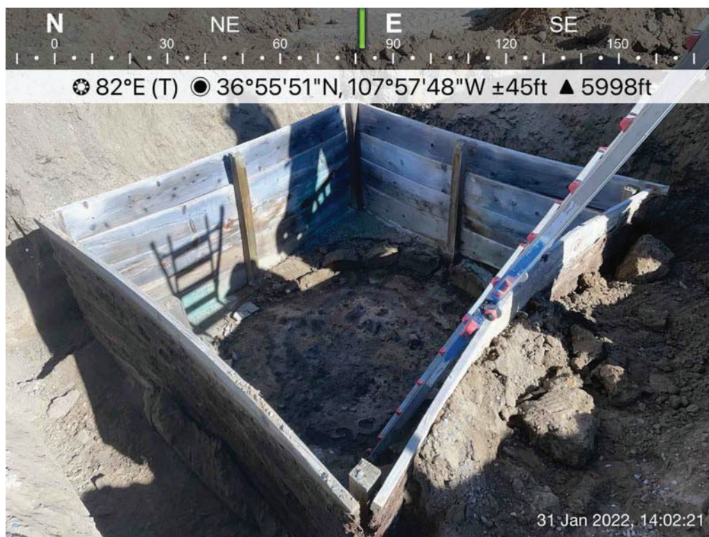
Photo 3: Former location of 45 bbls steel tank following removal, 1/31/2022.
