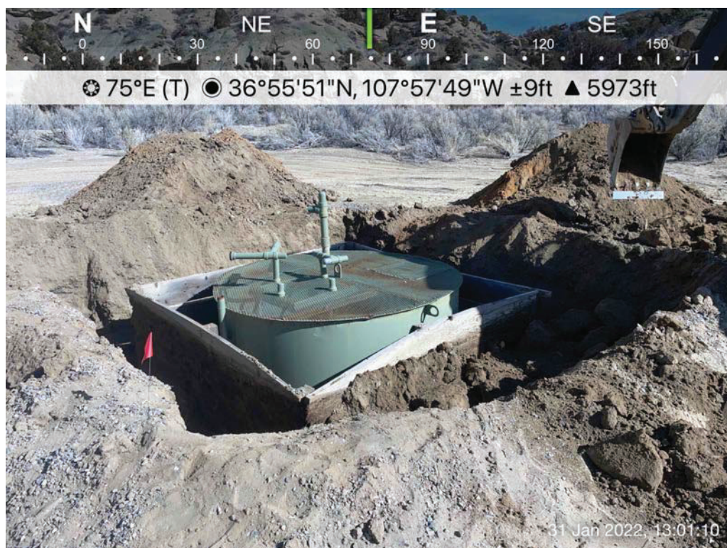
Photo 2: 45 bbls steel tank prior to removal, 1/31/2022.
