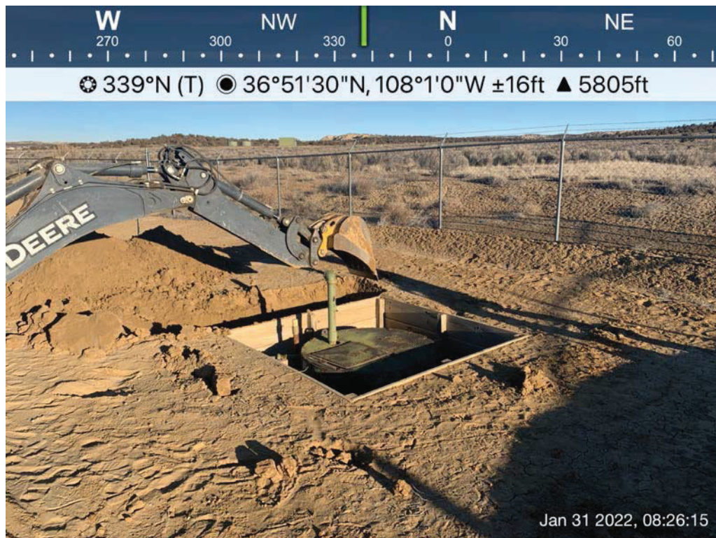
Photo 2: 21 bbls steel tank "B" prior to removal, 1/31/2022.
