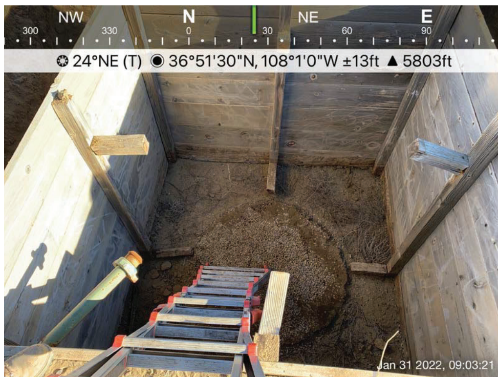
Photo 3: Former location of 21 bbls steel tank "B" following removal, 1/31/2022.
