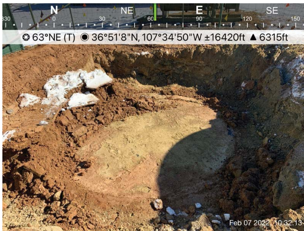
Photo 3: Former location of 40 bbls steel tank following removal, 2/7/2022.
