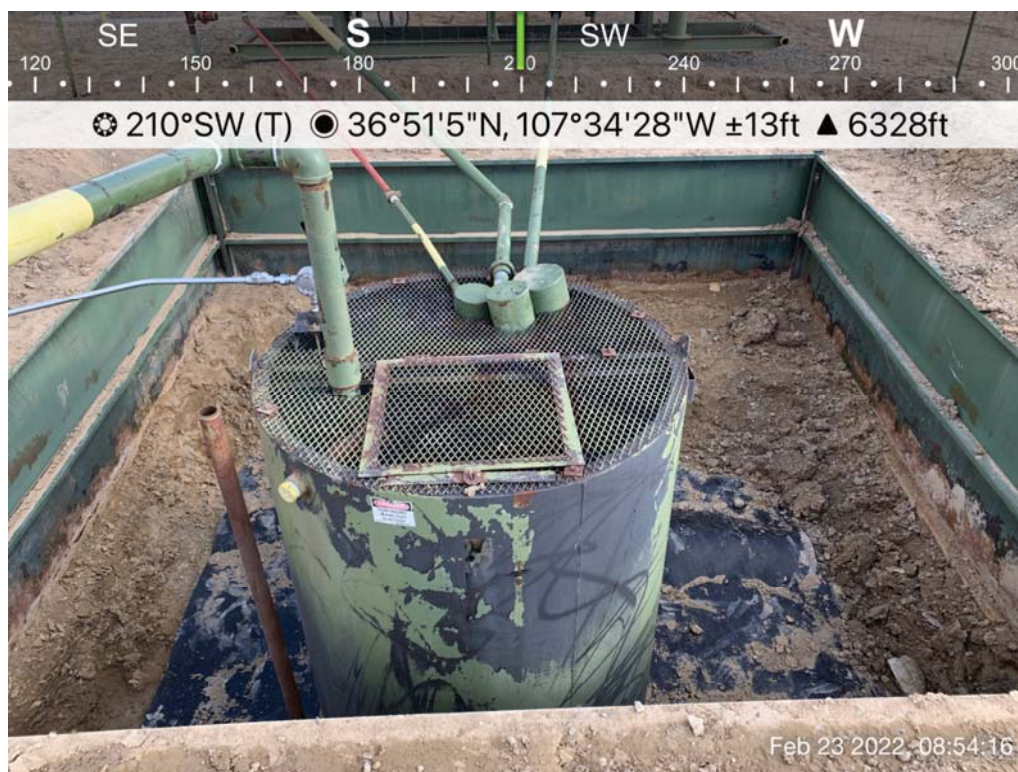
Photo 4: Replaced BGT with liner, 2/23/2022.
