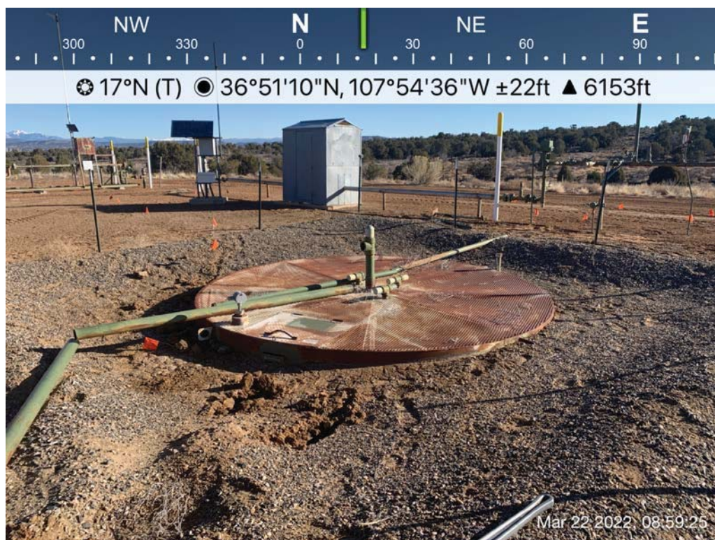
Photo 2: 95 bbls steel tank prior to removal, 3/22/2022.
