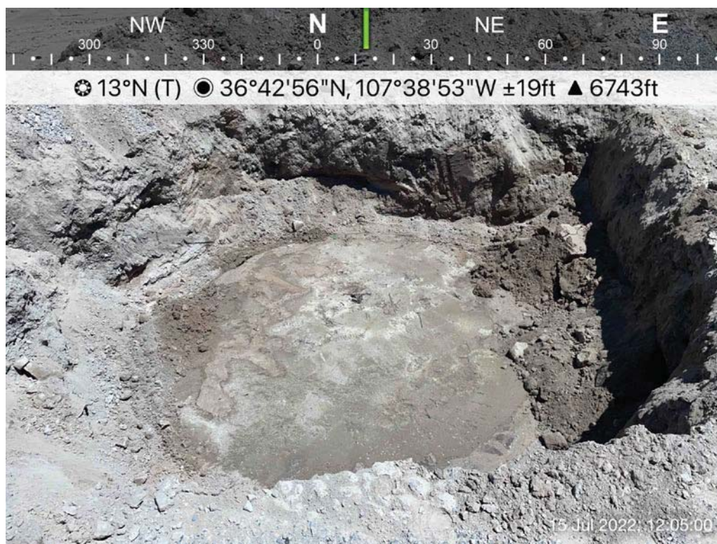
Photo 3: Former location of 95 bbls steel tank following removal, 7/15/2022.
