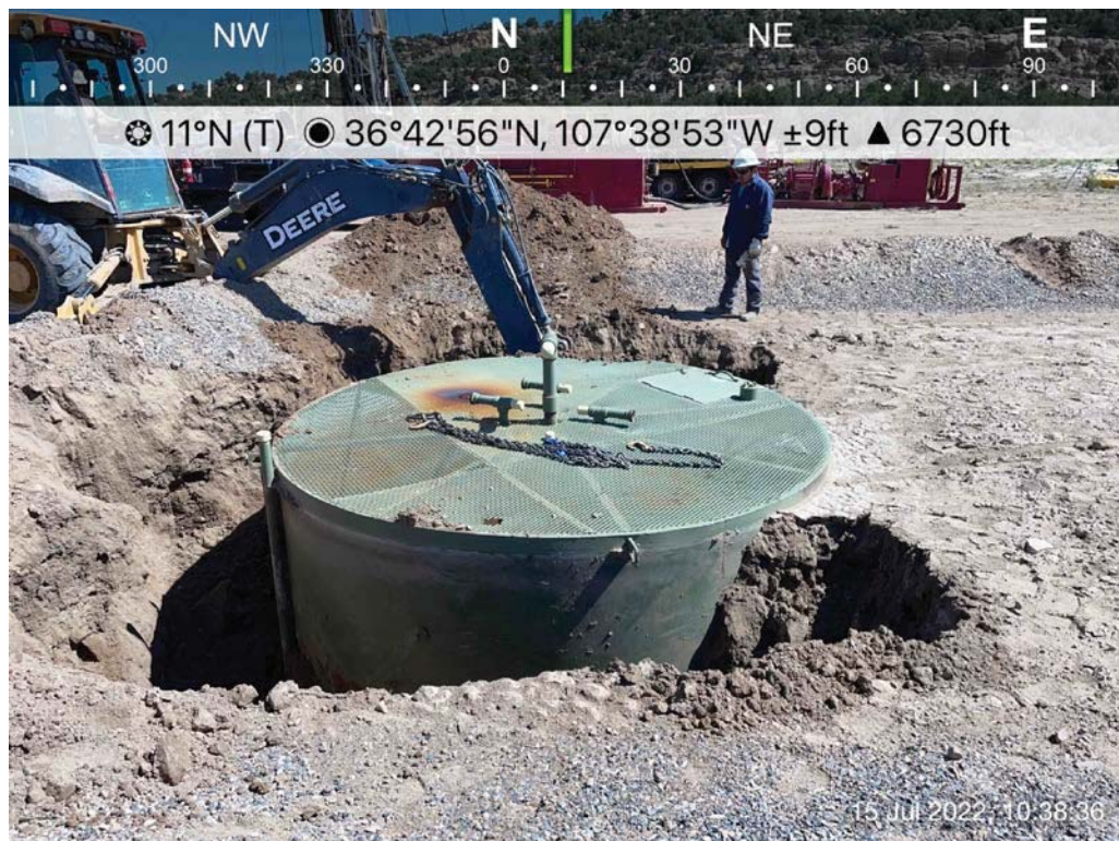
Photo 2: 95 bbls steel tank prior to removal, 7/15/2022.
