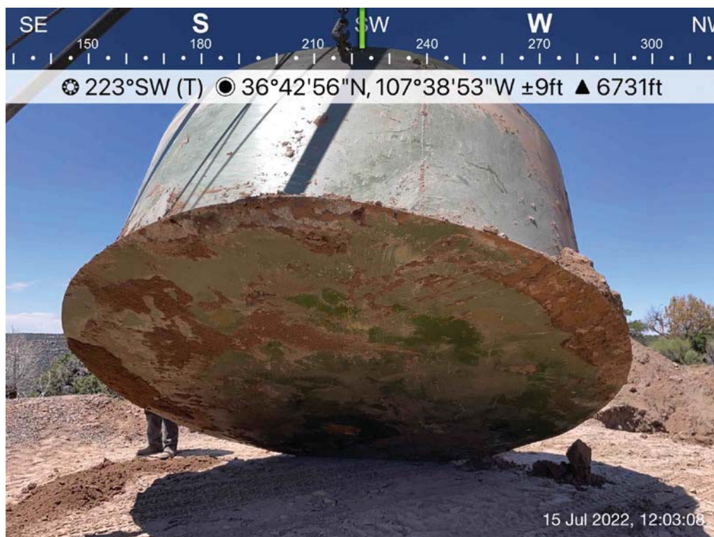
Photo 4: Bottom of steel tank following removal, 7/15/2022.
