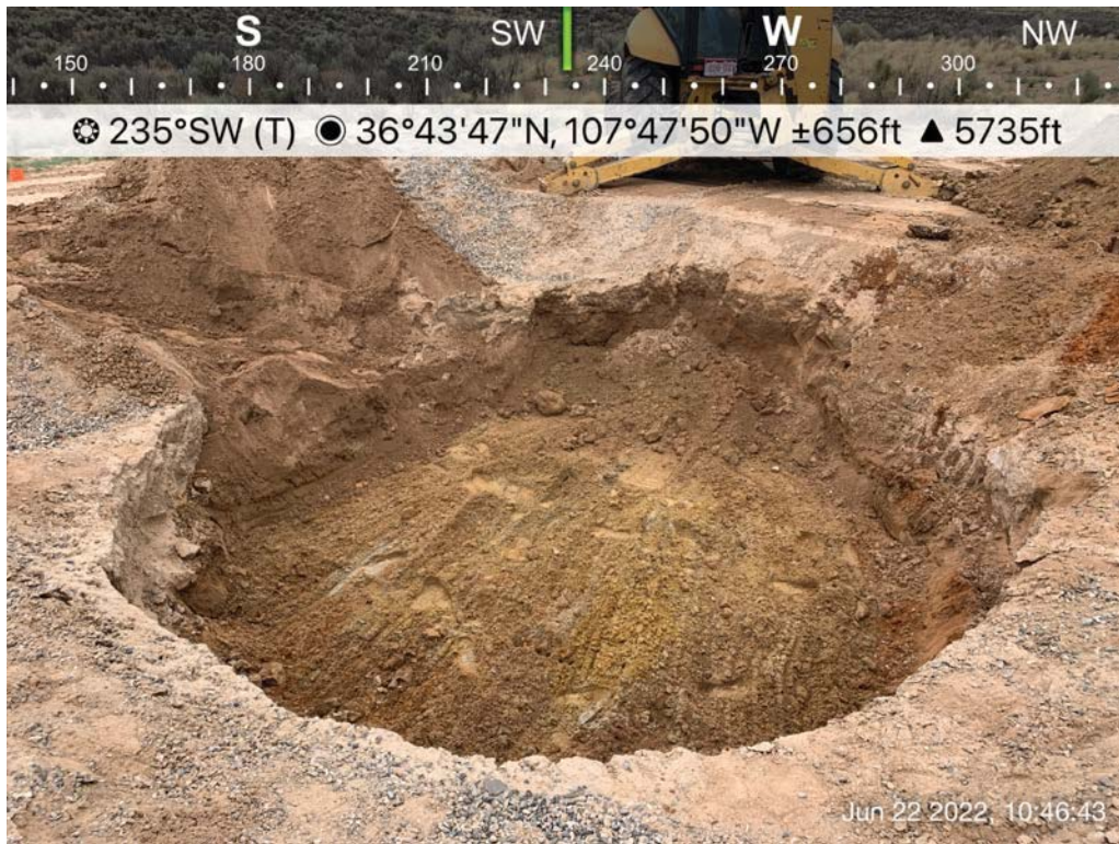
Photo 5: Former location of steel tank following excavation of additional soil and location of soil sample 5PC-TB@6'(95), 6/22/2022.
