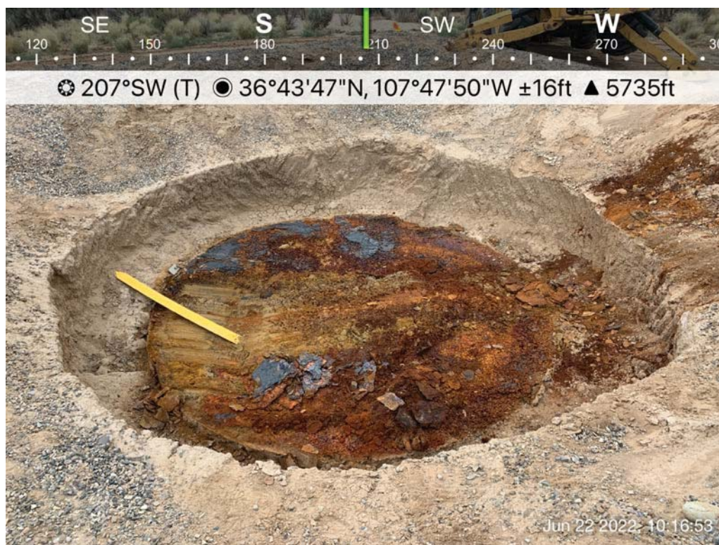
Photo 3: Former location of steel tank following removal and location of soil sample 5PC-TB@5'(95), 6/22/2022.
