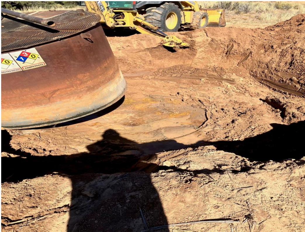
Photo 2: BGT Being Removed
