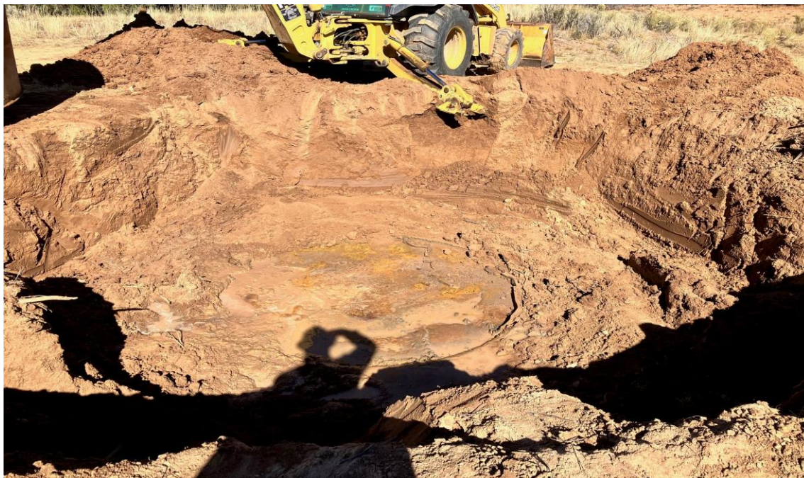
Photo 3: BGT Cellar After Removal
