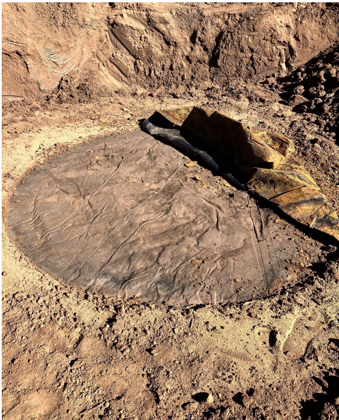
Photo 3: BGT Cellar After Removal with Liner Pulled Back
