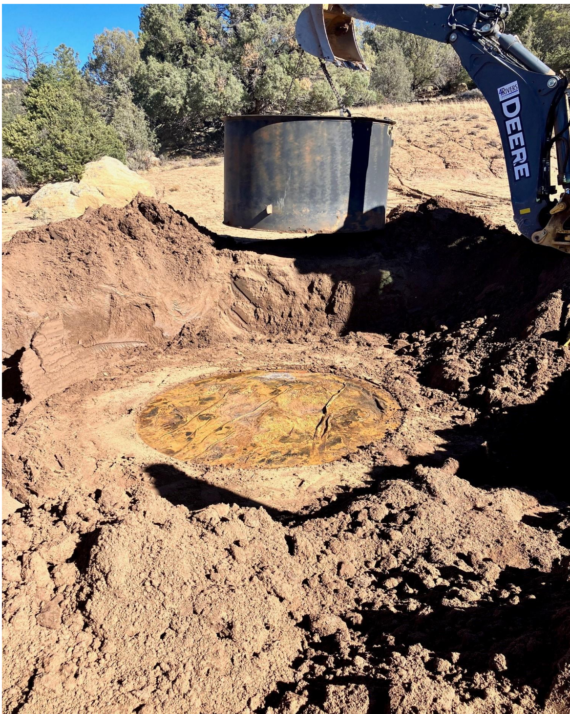
Photo 2: BGT Being Removed with Liner in Bottom of Cellar
