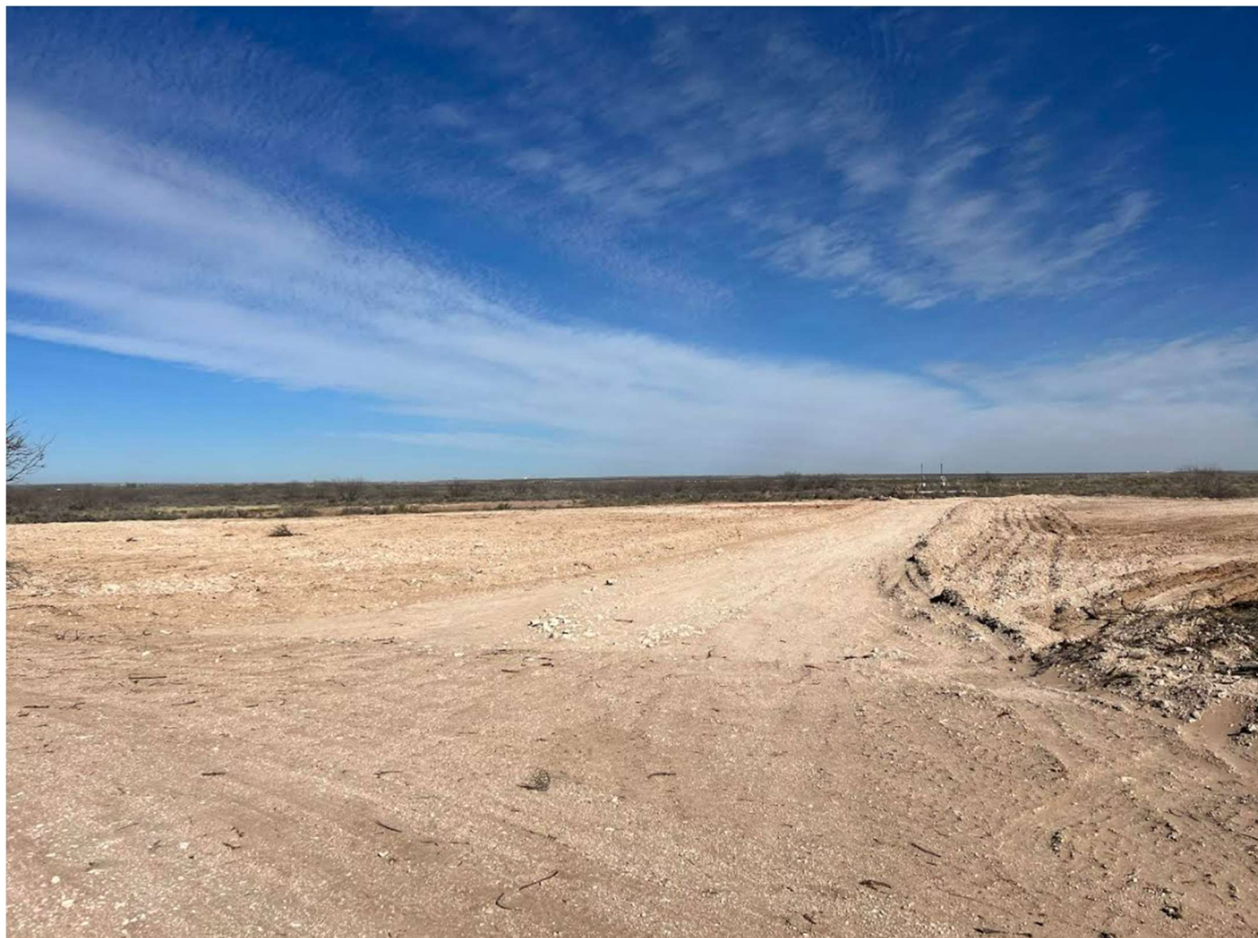
Figure 2: Pad caliche removed and seeded
