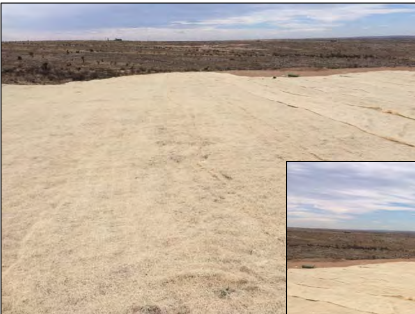
Erosion control blanket over backfilled surface 3/9/2018
