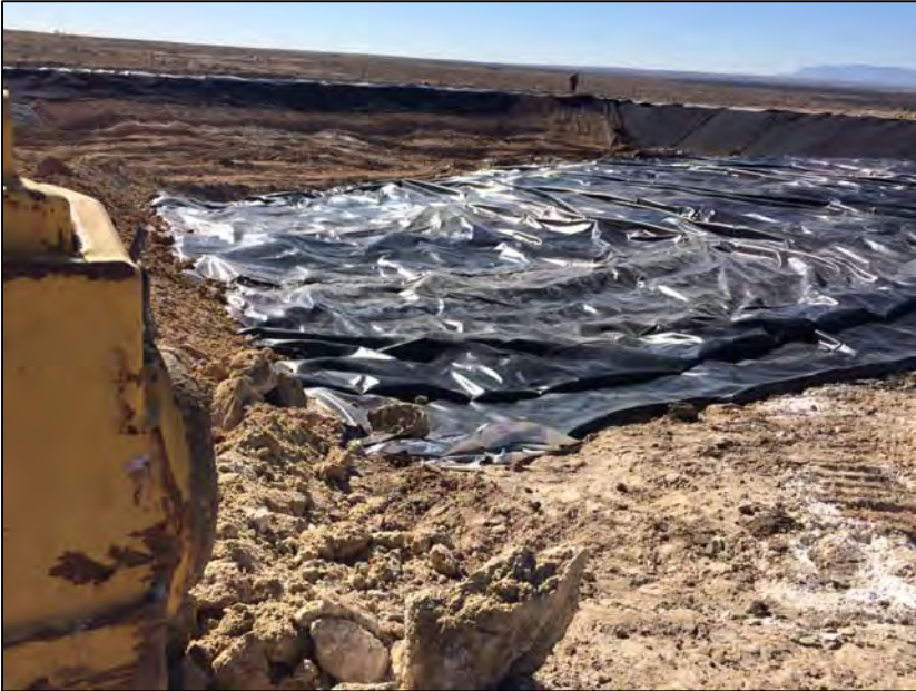
Installing liner over cuttings and backfilling 12/13/2017
