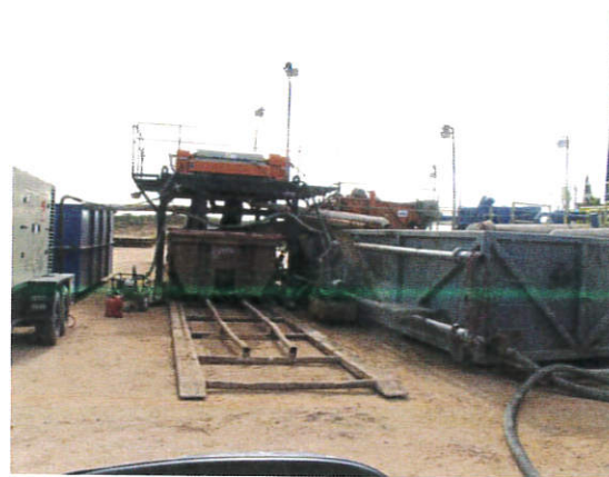
Above: Centrifugal Closed Loop System
