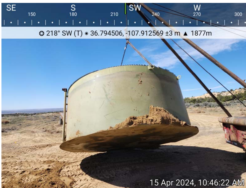
Photo 4: Bottom of BGT following removal, 4/15/2024.
