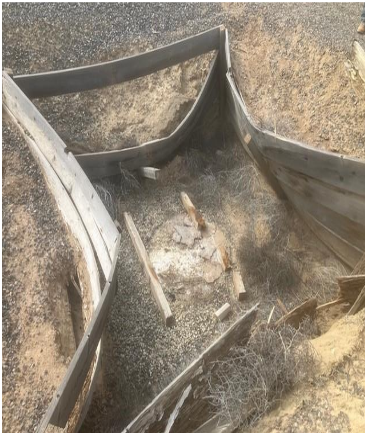
Photo 3: BGT Cellar after Tank Removal
