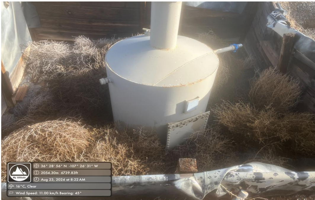
Photo 2: BGT in Cellar
