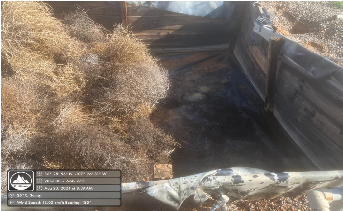
Photo 3: BGT Cellar after Tank Removal
