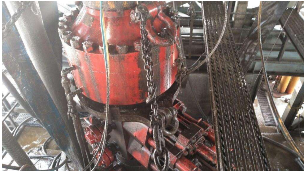
Figure 1: Winch System attached to BOP Stack
