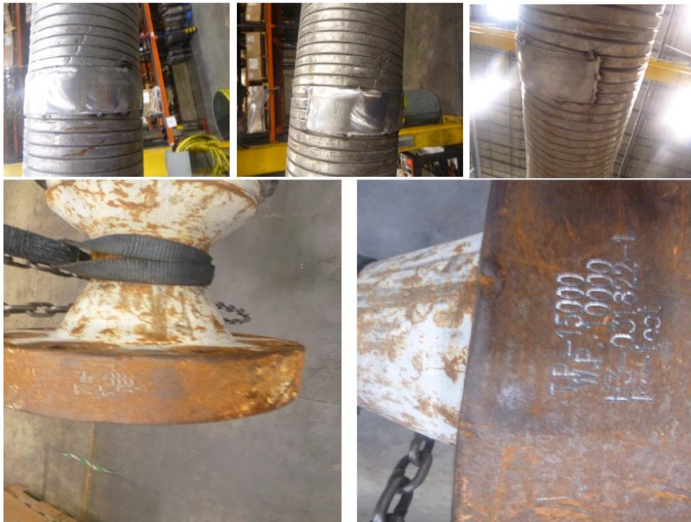
Photos: Repaired Armor and Engraving.
