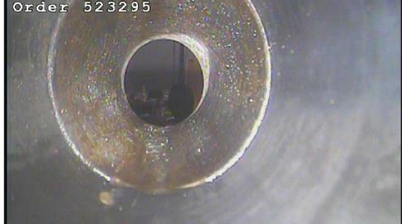
Photos: Liner/Coupling Interface END 2
