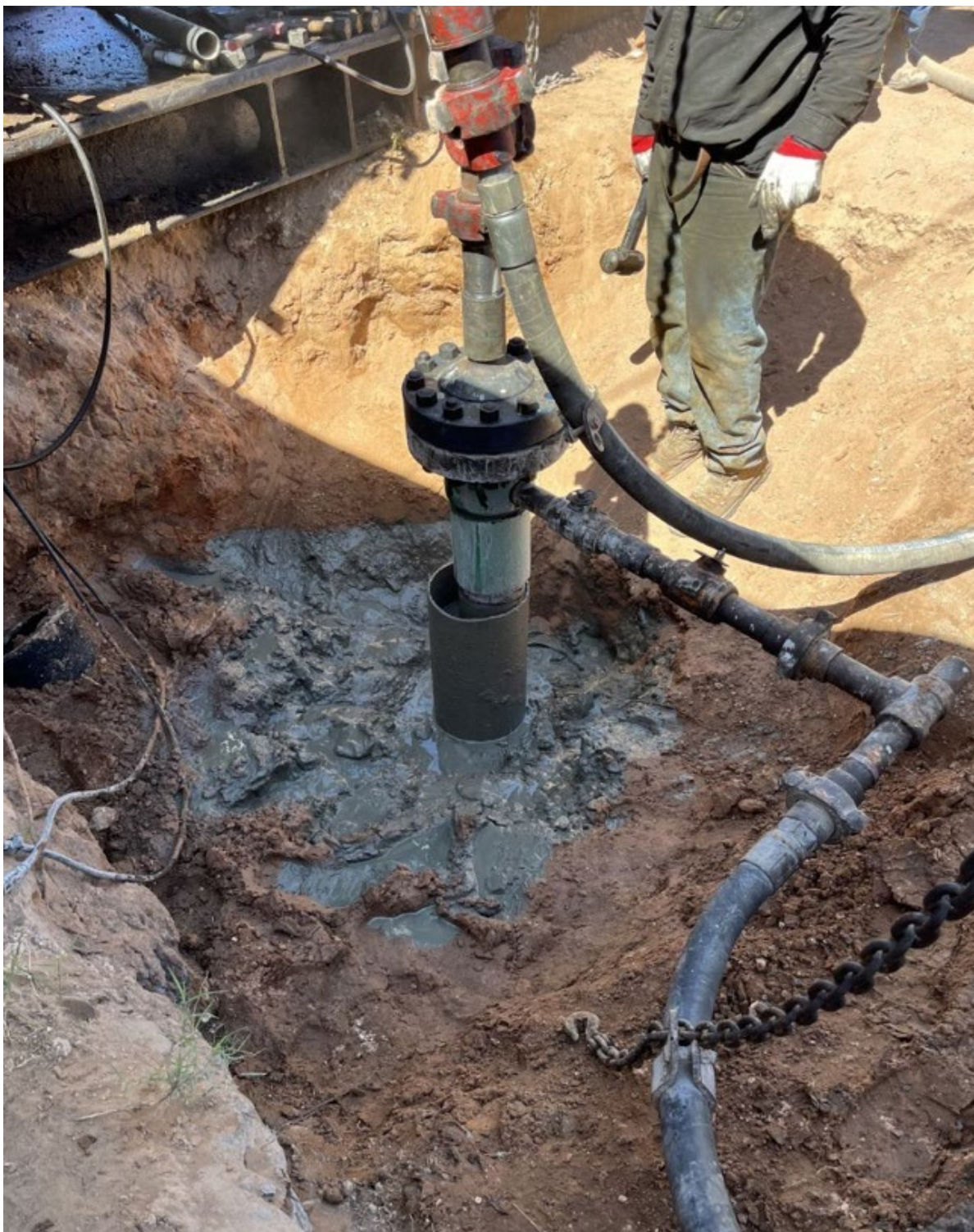
Figure 4: 9/29/24 Pumping cement down the 7" casing
