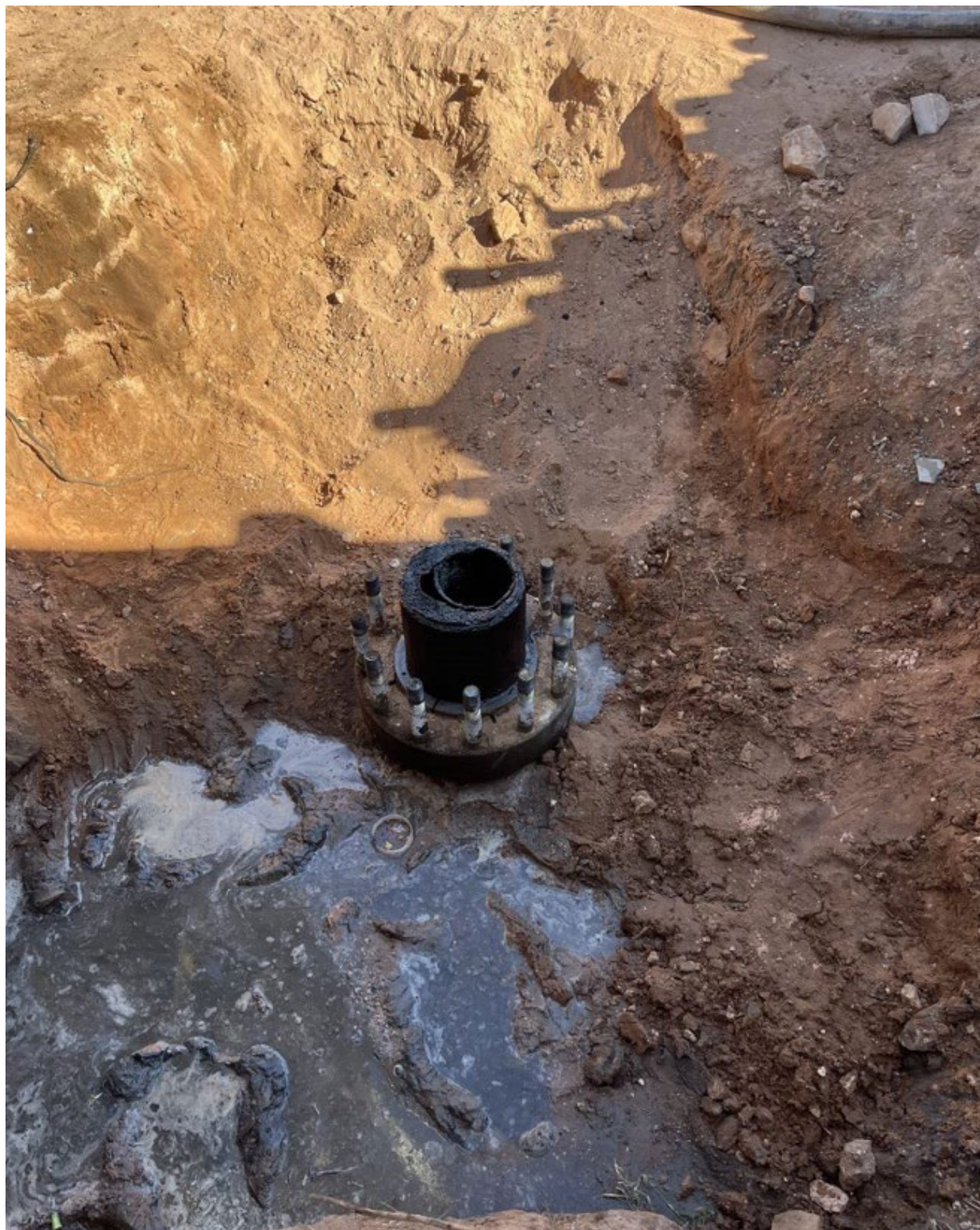
Figure 3: BOP & top half of slip-on adapter removed from the 10.75" casing. The 10.75" and 7" casings are exposed.
