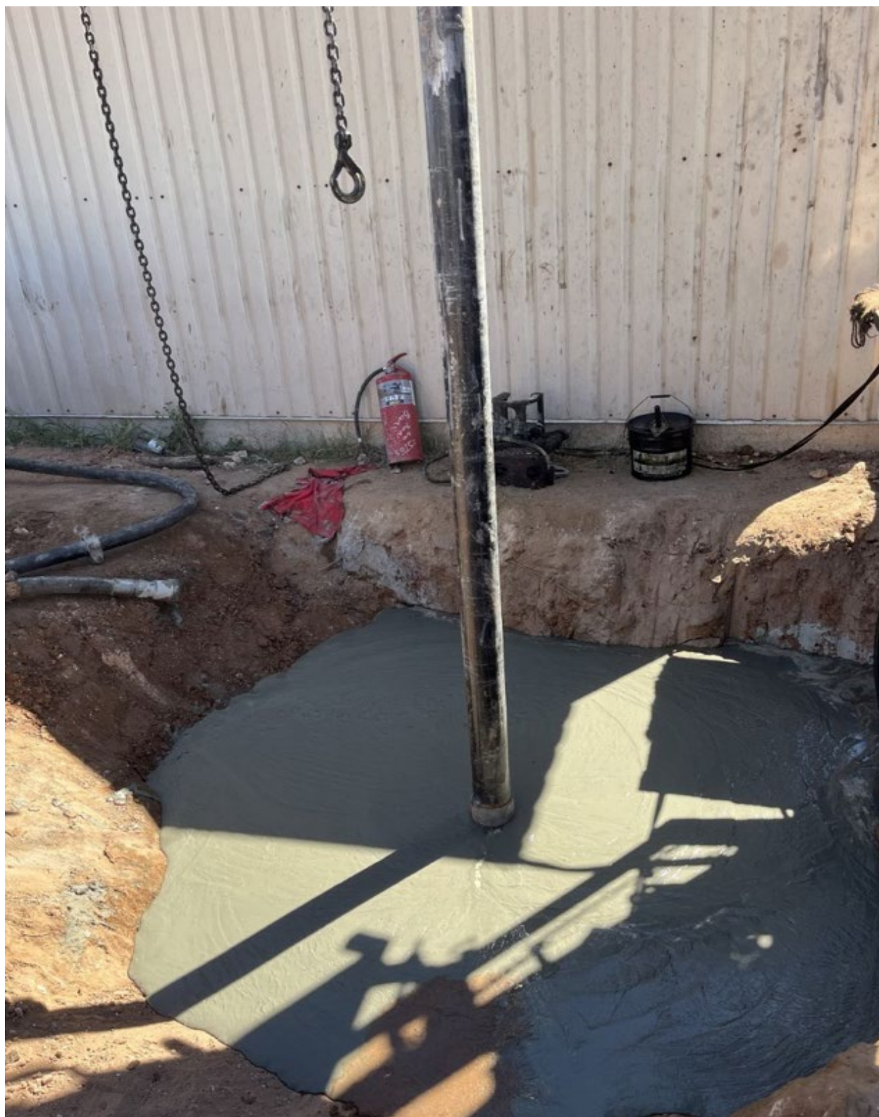
Figure 6: 9/29/24 Dry hole marker installed, well is plugged and abandoned
