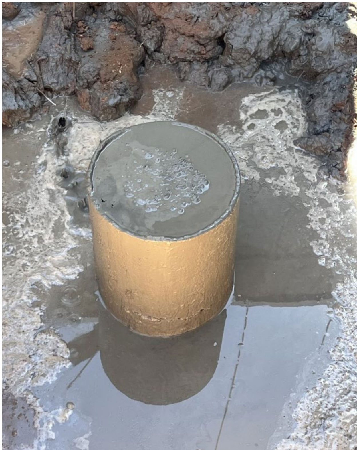
Figure 5: 9/29/24 Both the 7" and 10.75" casings filled with cement
