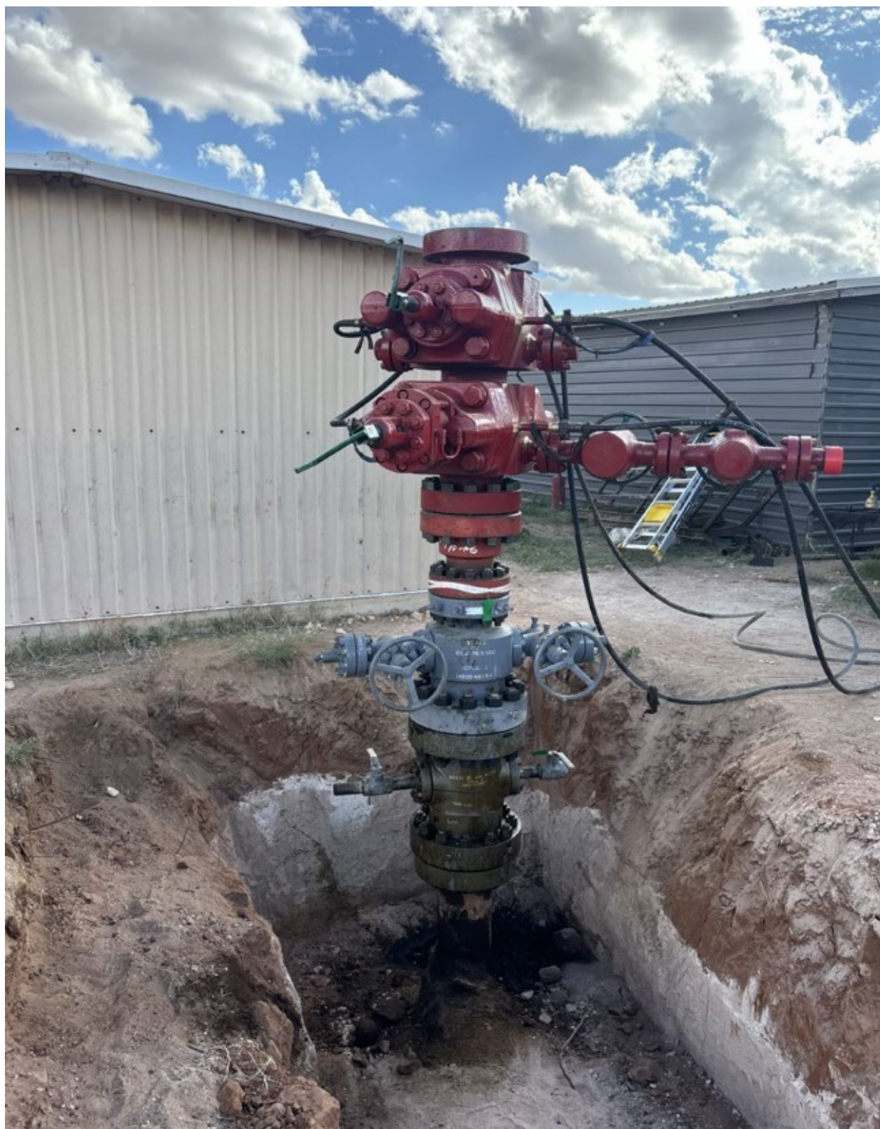
Figure 2: 9/16/24 Wellhead and BOP installation achieved
