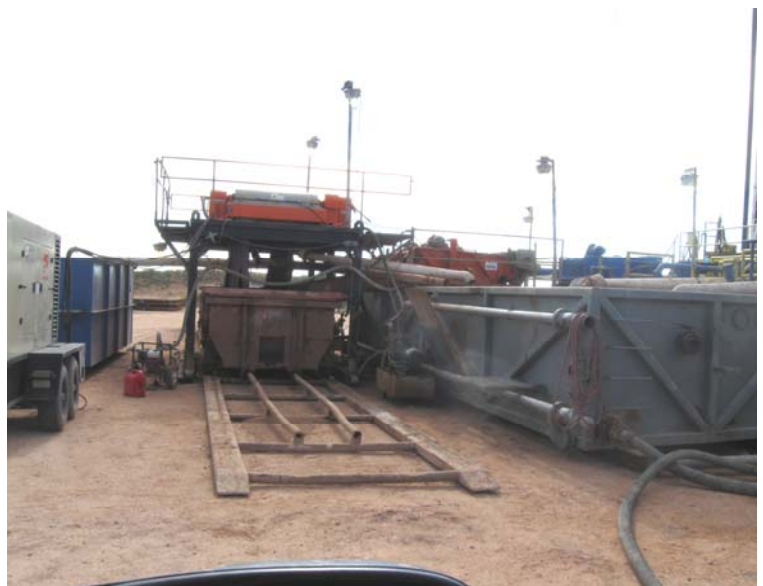
Above: Centrifugal Closed Loop System
