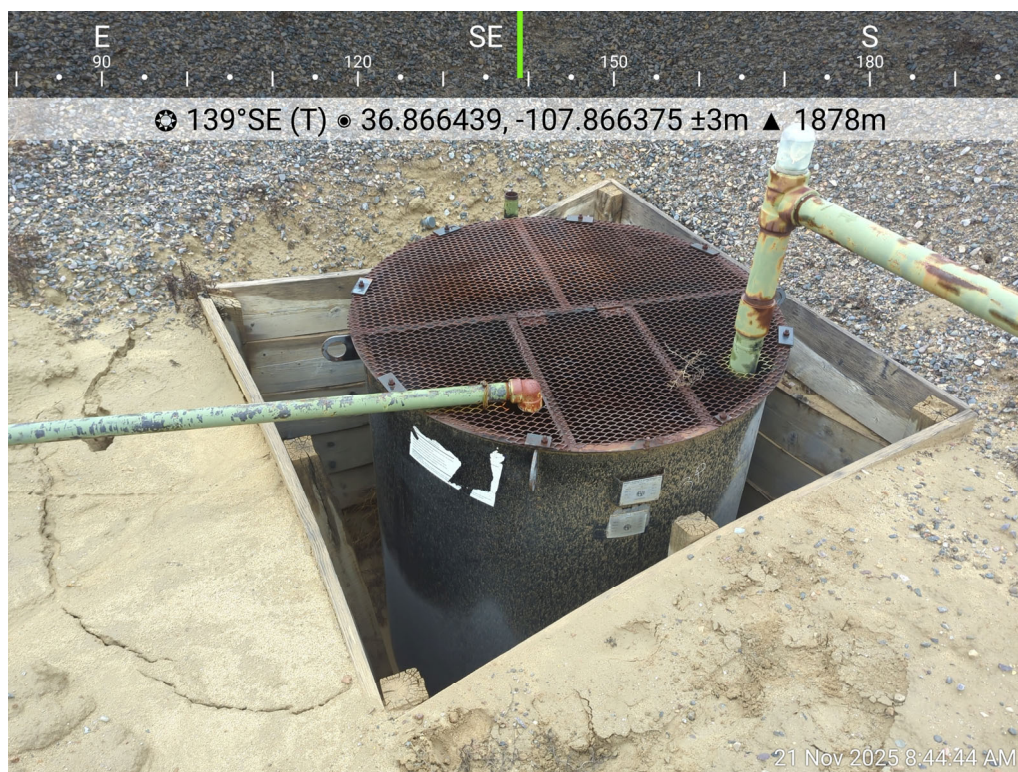
Photo 2: BGT prior to removal.
