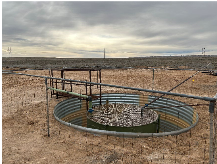
Photo 2-4: After installation of new BGT
