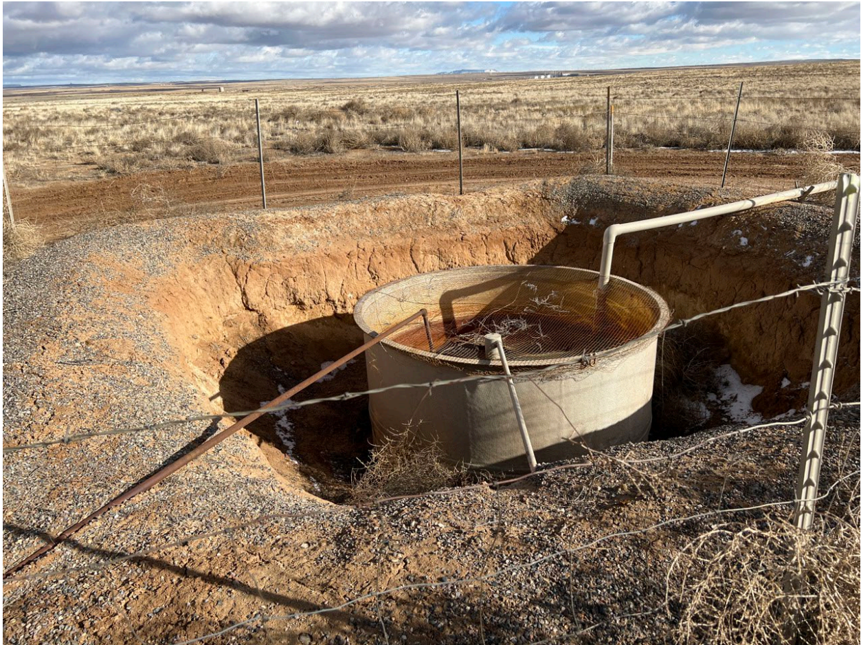
Photo 1: BGT Before Remediation
