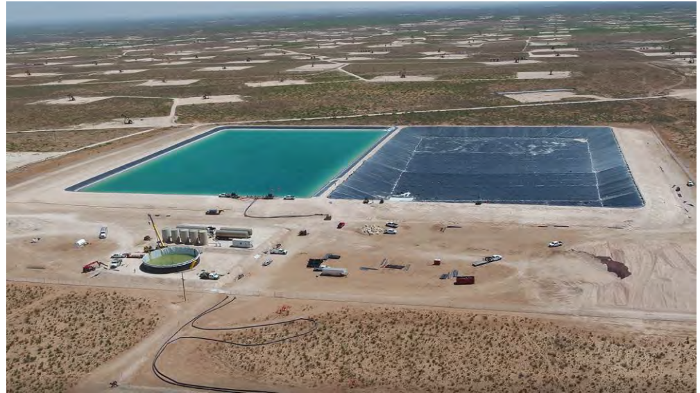
Image: Longfellow's 2MMBbl Produced Water Recycling & Storage Facility
