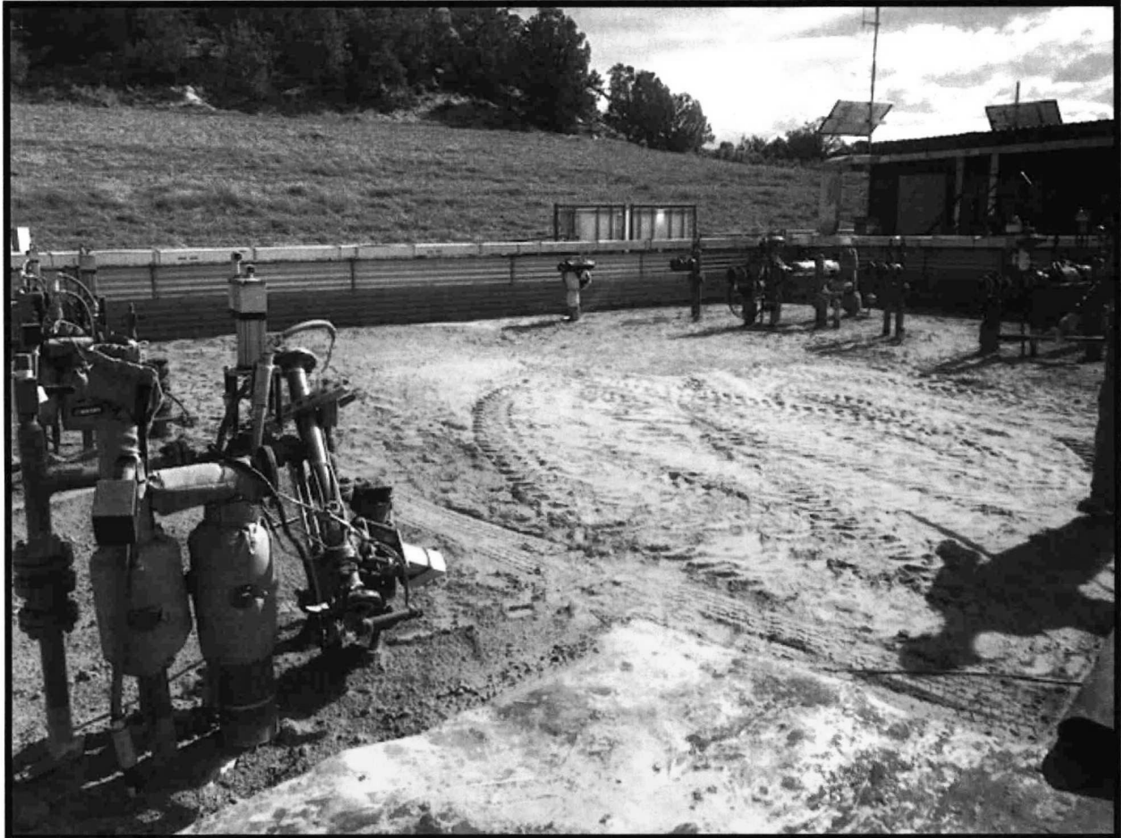
Photo: Area Back Filled
