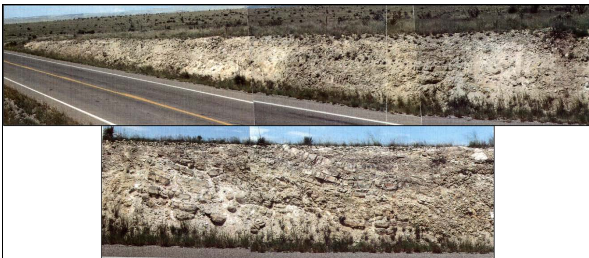
Figure B26. San Andres collapse breccia along U.S. Highway 82 near the foothills of the Sacramento Mountains, New Mexico. Meteoric recharge dissolved San Andres evaporite strata ( \text{CaSO}_4 ), which caused carbonate strata forming the roof to collapse. Dissolved evaporite strata ( \text{CaSO}_4 ) added sulfate ( \text{SO}_4 ) to low salinity ( <10,000 ppm) meteoric water as it recharged into the subsurface.
