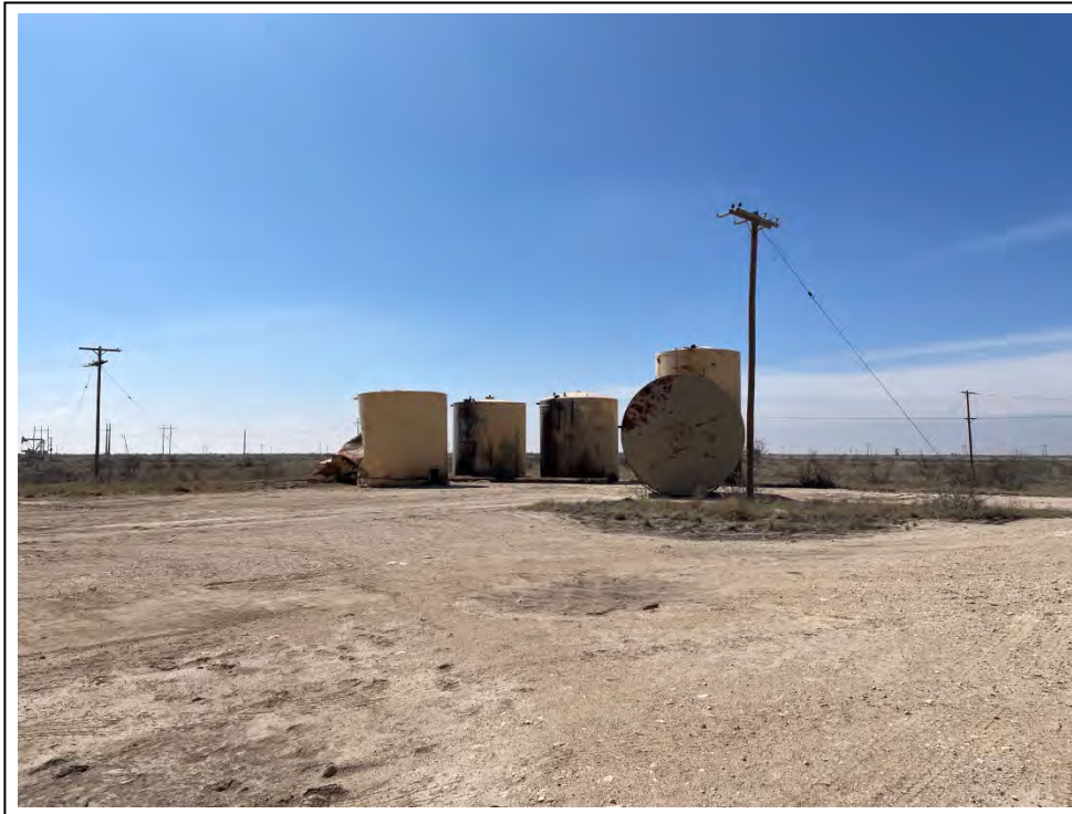
1. Empty ASTs staged for removal
