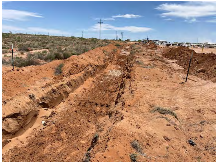
Photograph 7: View of central excavation area facing south.
