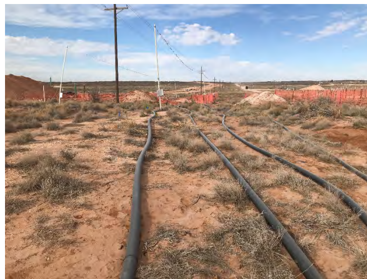
Photograph 4: View of southern release extent facing north.
