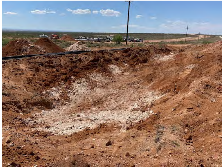
Photograph 5: View of southern excavation area facing north.
