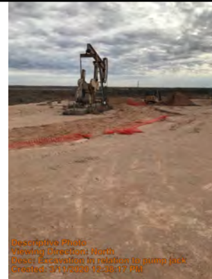
Excavation in relation to pump jack
