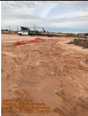
Length of excavation
