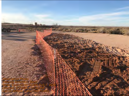
Viewing Direction: West
