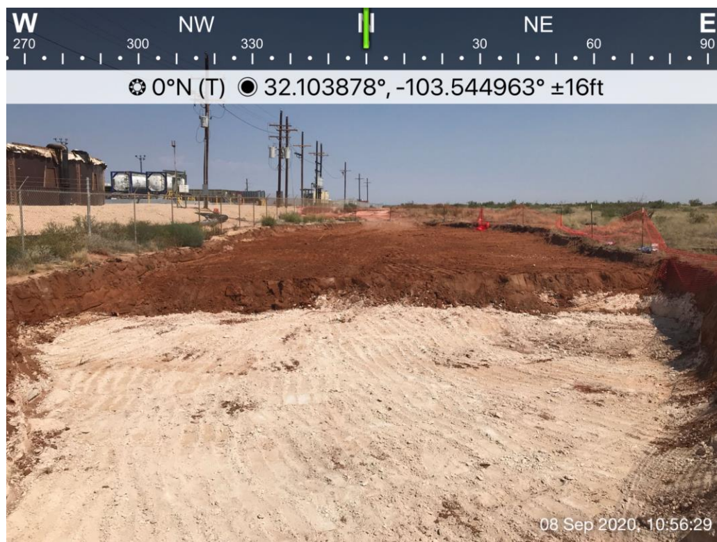
View North, areas of excavation Bottom Holes (1 – 34)
