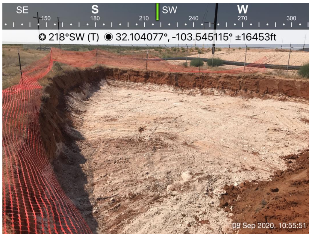
View South, areas of west Bottom Holes (26 – 34)
