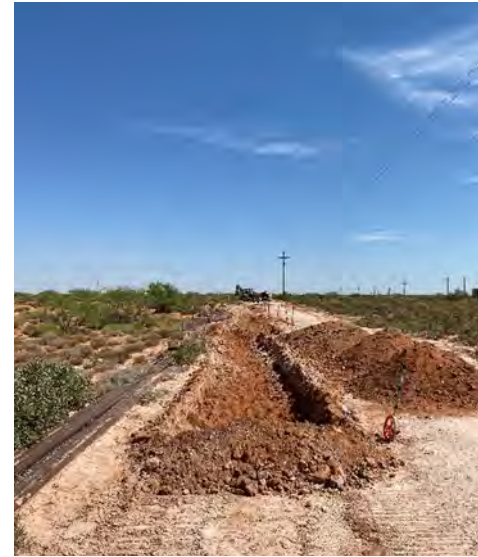
Photograph 6: Excavation extent on lease road facing North
