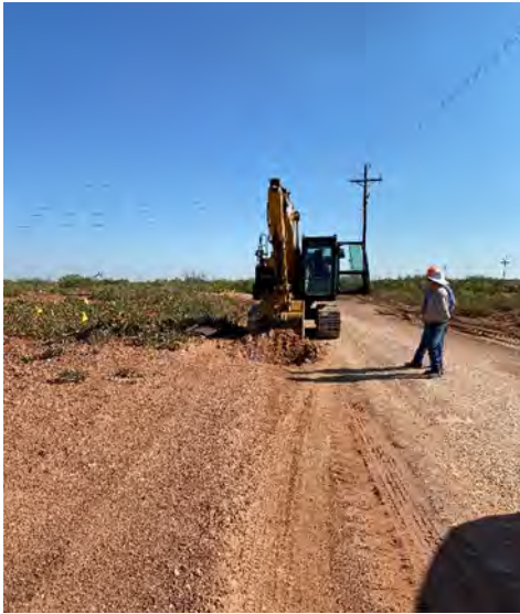
Photograph 5: Delineation of release extent via trackhoe facing North
