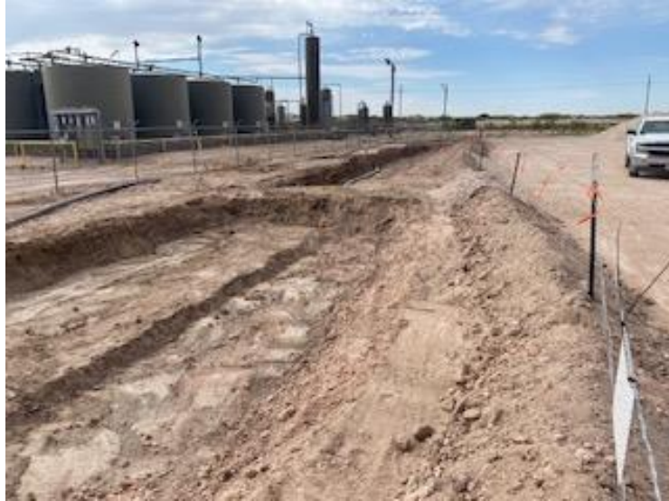
Photograph 13: Southeast view of the excavation.
