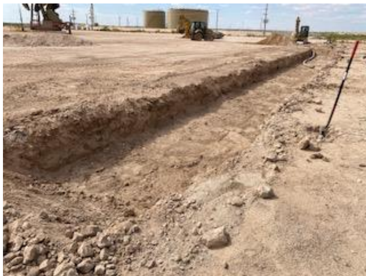
Photograph 9: Excavation activities in the southern release area.
