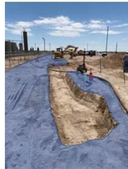
Photograph 16: Northern portion of the deferral area in blue, viewing south.
