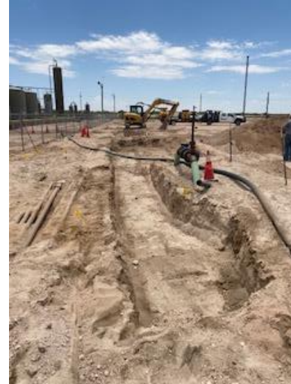
Photograph 14: Northern portion of the excavation, viewing south.
