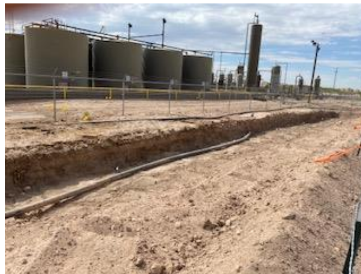
Photograph 12: Final southern excavation extent.
