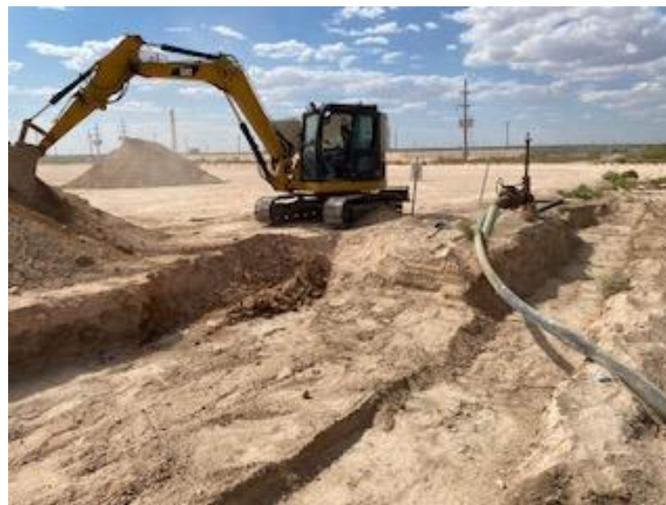
Photograph 10: Excavation activities in the northern release area.
