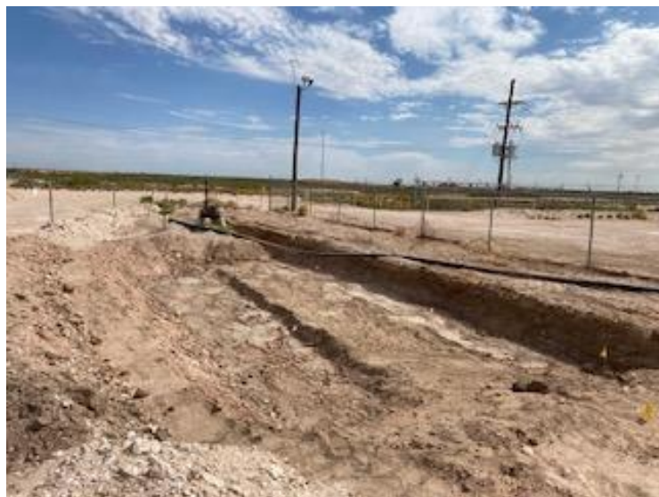
Photograph 11: Final northern excavation extent.
