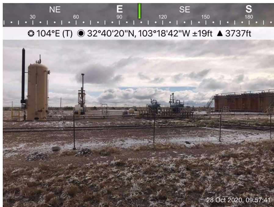
Impacted area viewing east, October 28, 2020
