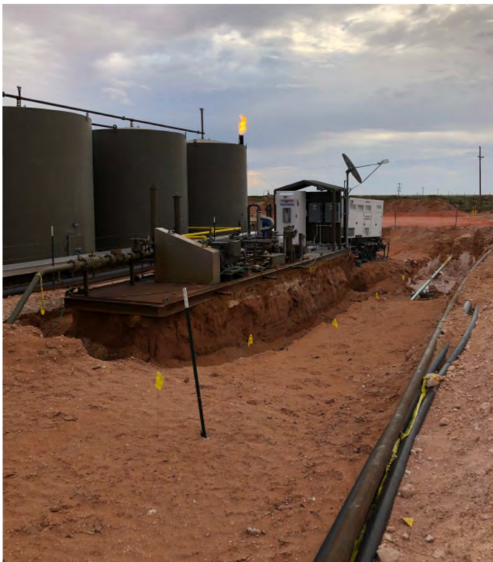
Photo 2 August 19, 2020 View of foundation failing in the area of Sample WT-Comp-2.
