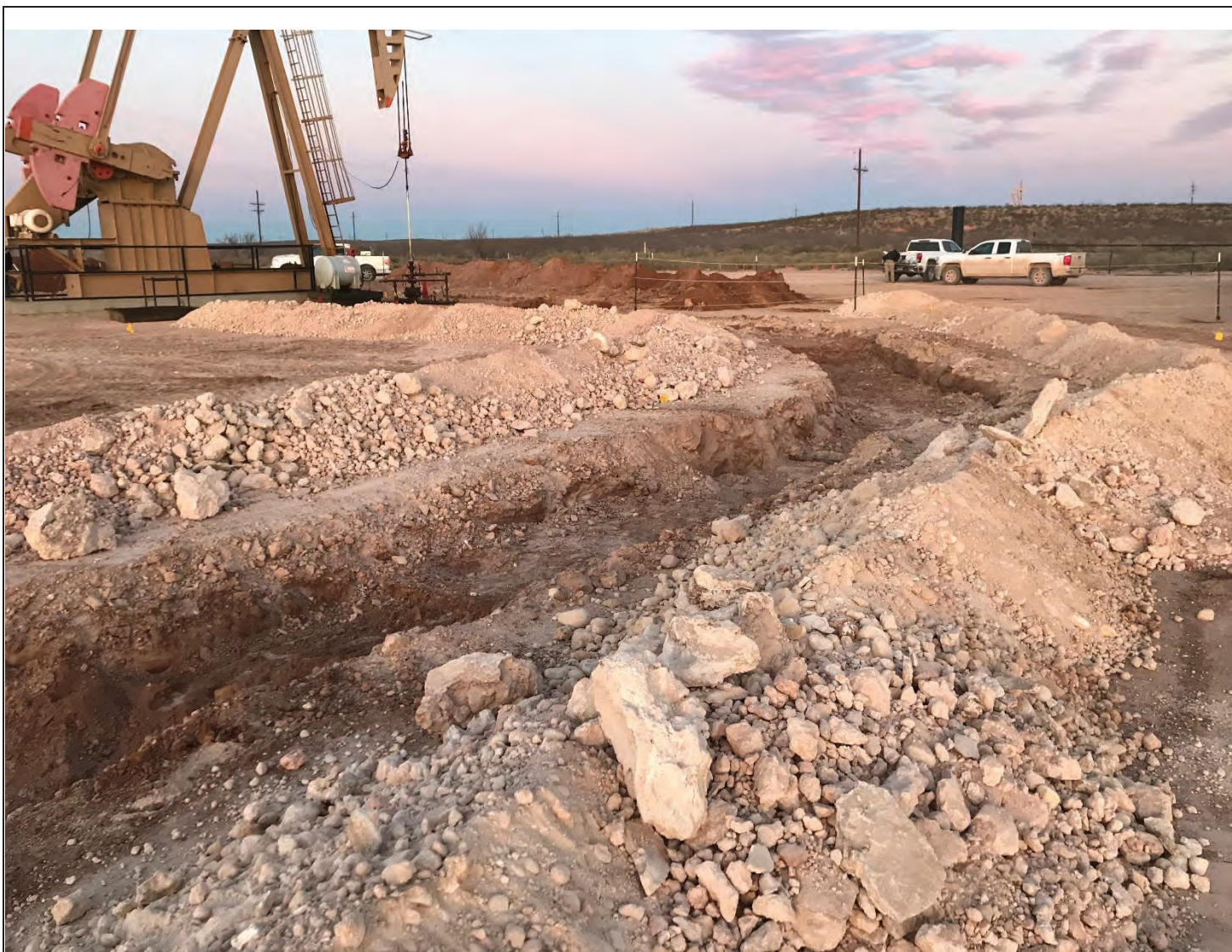
Eastern view of the excavation area.
