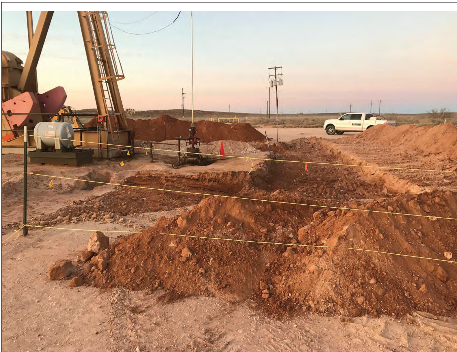
Western north of excavation area.
