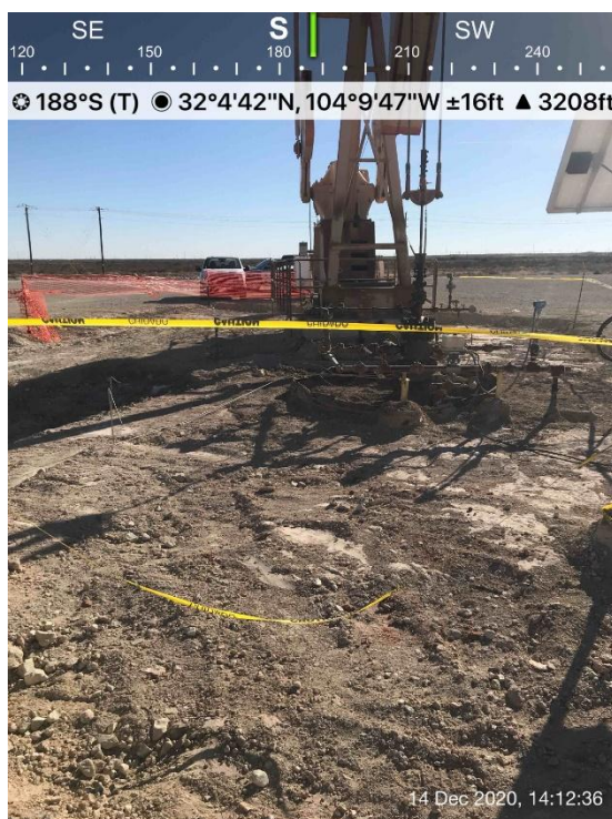
Excavated soil viewing south, December 14, 2020
