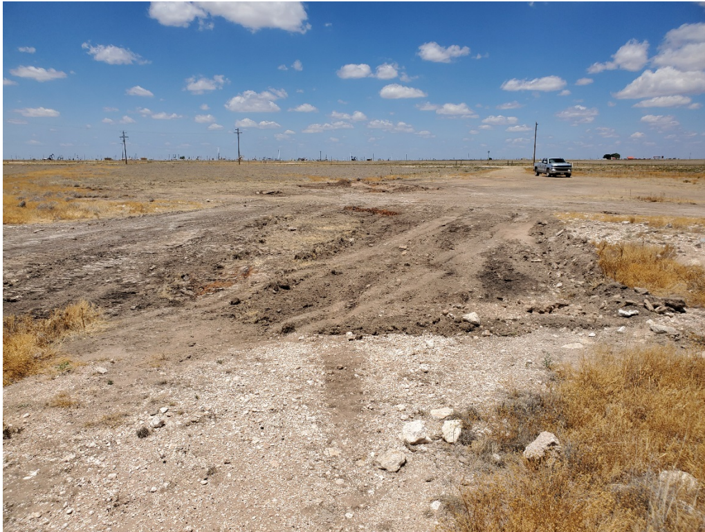
Spill area partially excavated
