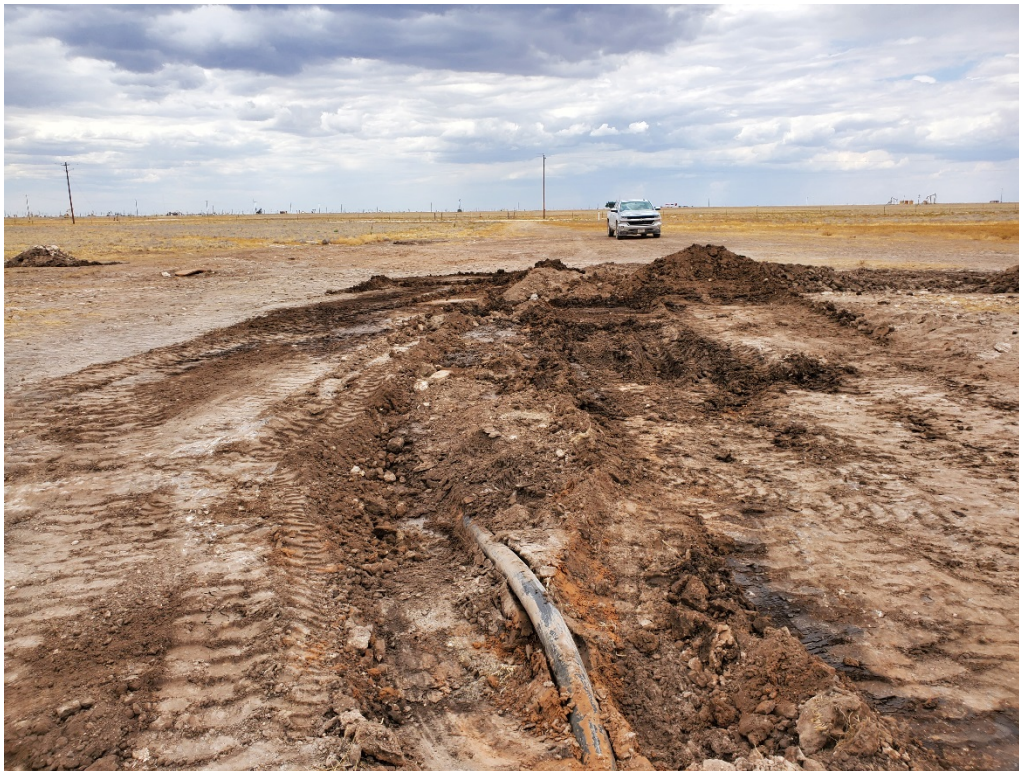
Spill area excavated.
